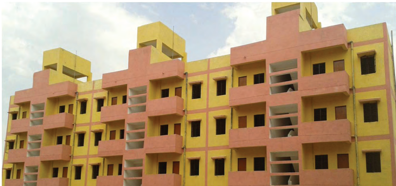
EWS Housing under JNNURM-VGF at Jabalpur, Madhya Pradesh
