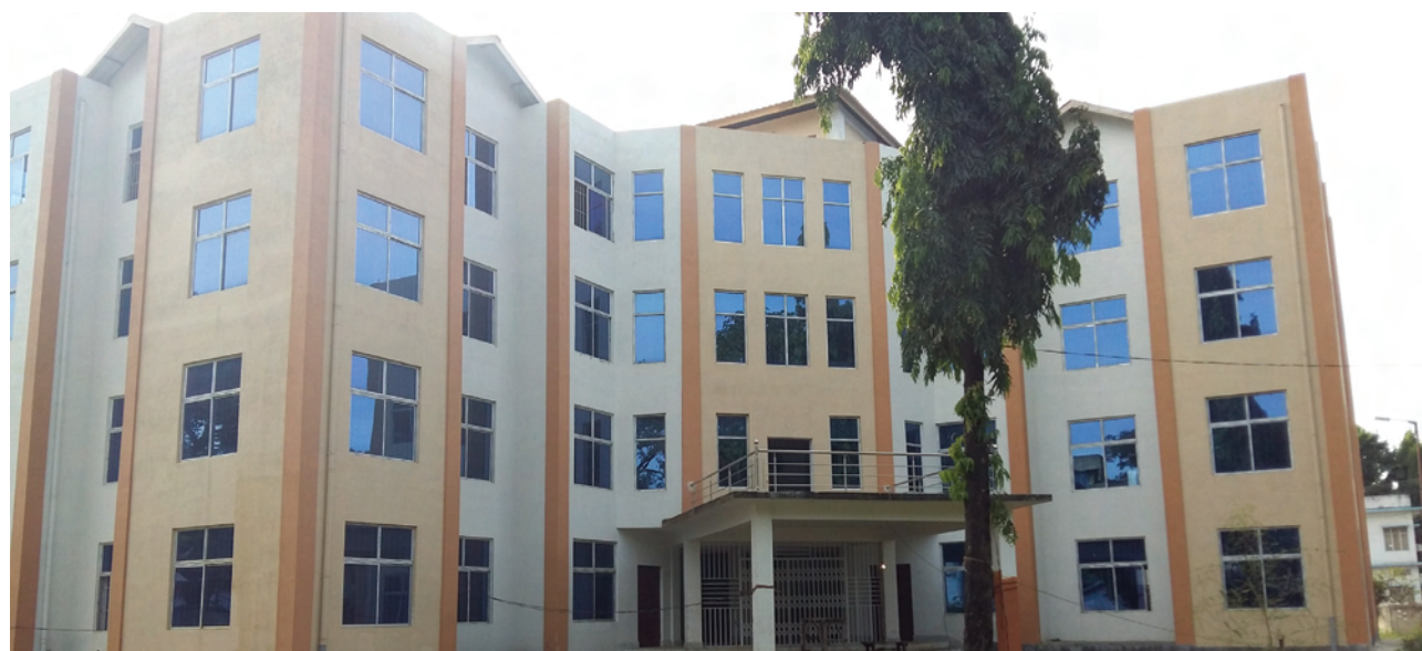
HUDCO Financed PWD Office Complex Dimapur, Nagaland
