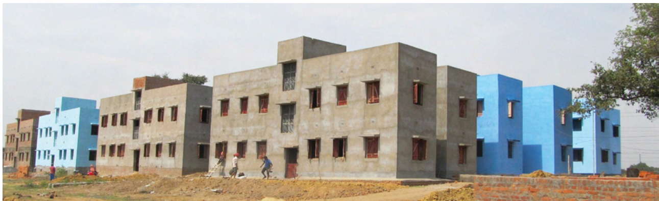
BSUP Block Housing at Asansol, West Bengal
