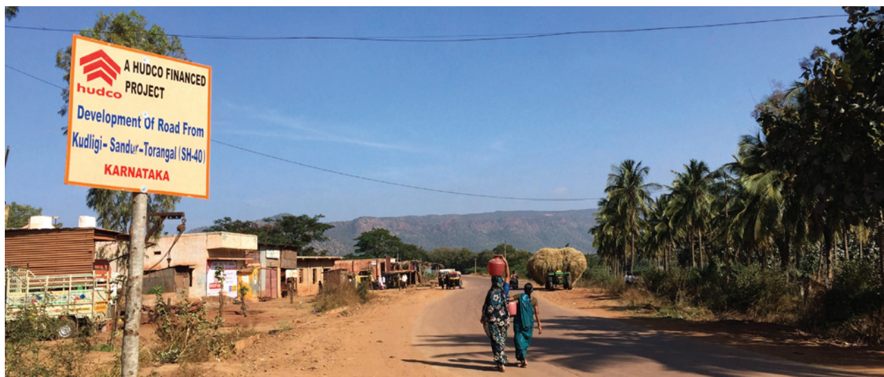
HUDCO financed road project at Bellary, Karnataka
