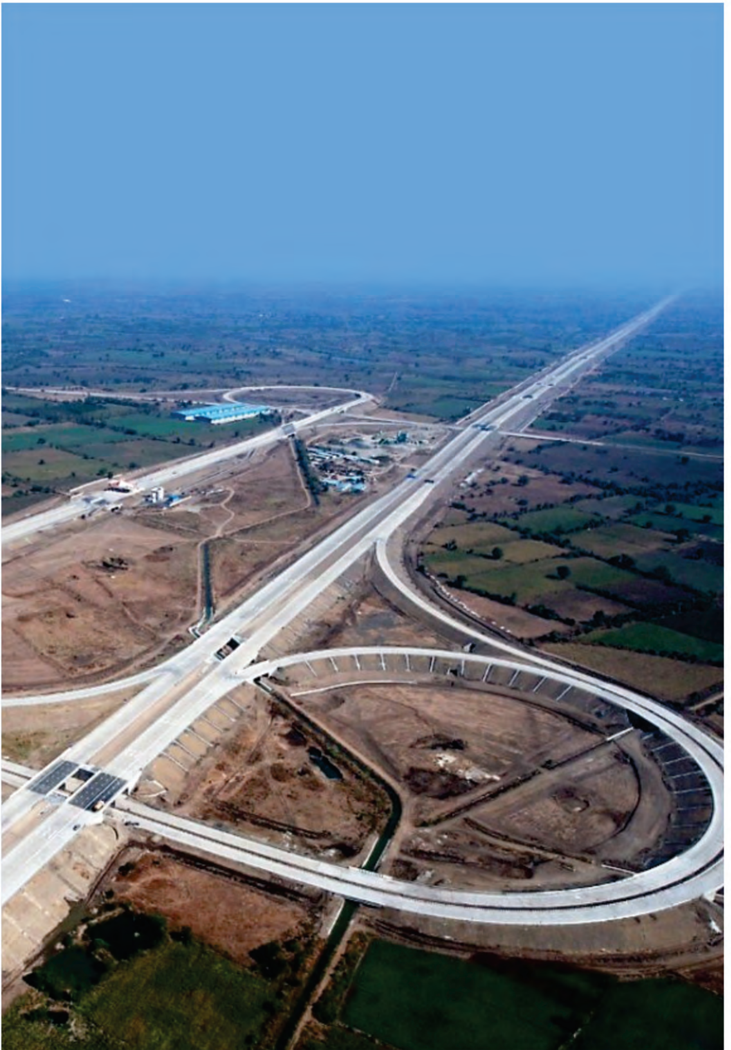
Dhamangaon Interchange, Nagpur-Mumbai Super Communication Expressway, Maharashtra
