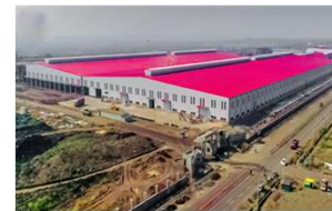
Pre-engineered Steel Buildings
