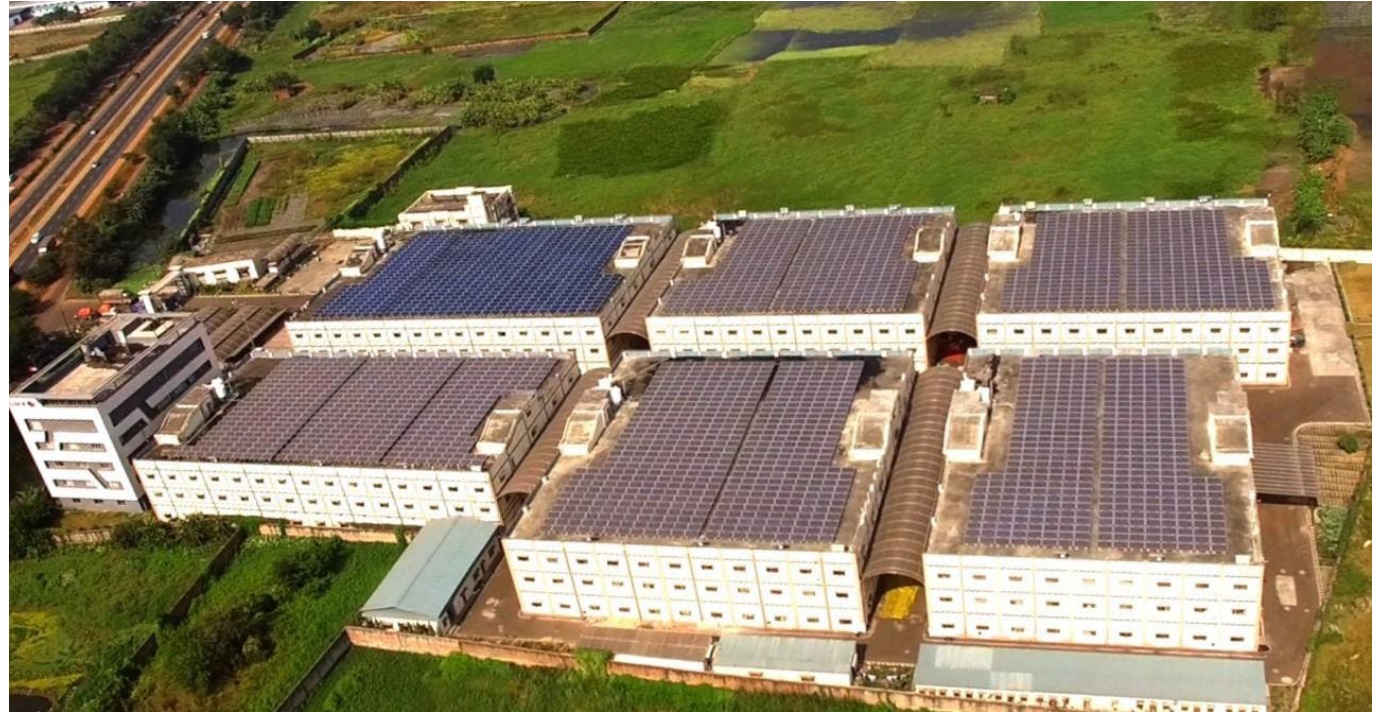
Rooftop solar power plant at Dankuni unit
