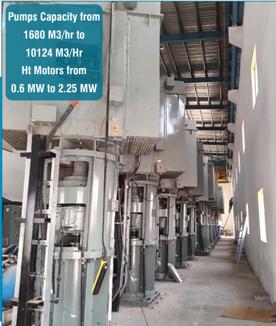
NVDA KHALWA LIFT MICRO IRRIGATION PROJECT 30 Nos Large Capacity Pumps and HT Motors
