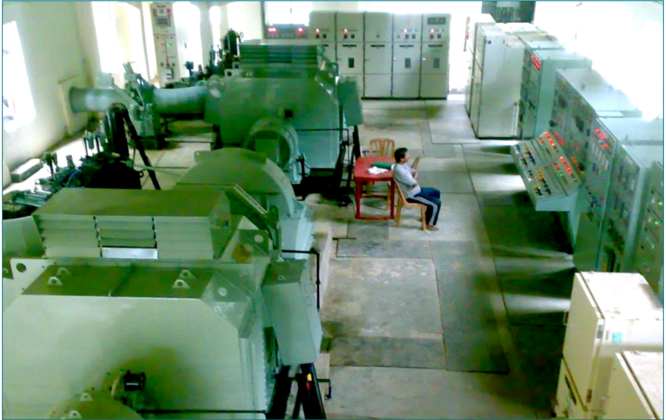
2 X 1500KW MAICHEM PHASE II HORIZONTAL TURGO IMPULSE TURBINE WITH GENERATOR GOVERNMENT OF MIZORAM
