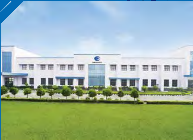
Aluminium Die Casting, Suspension & Braking Systems Plant, Pantnagar, India
