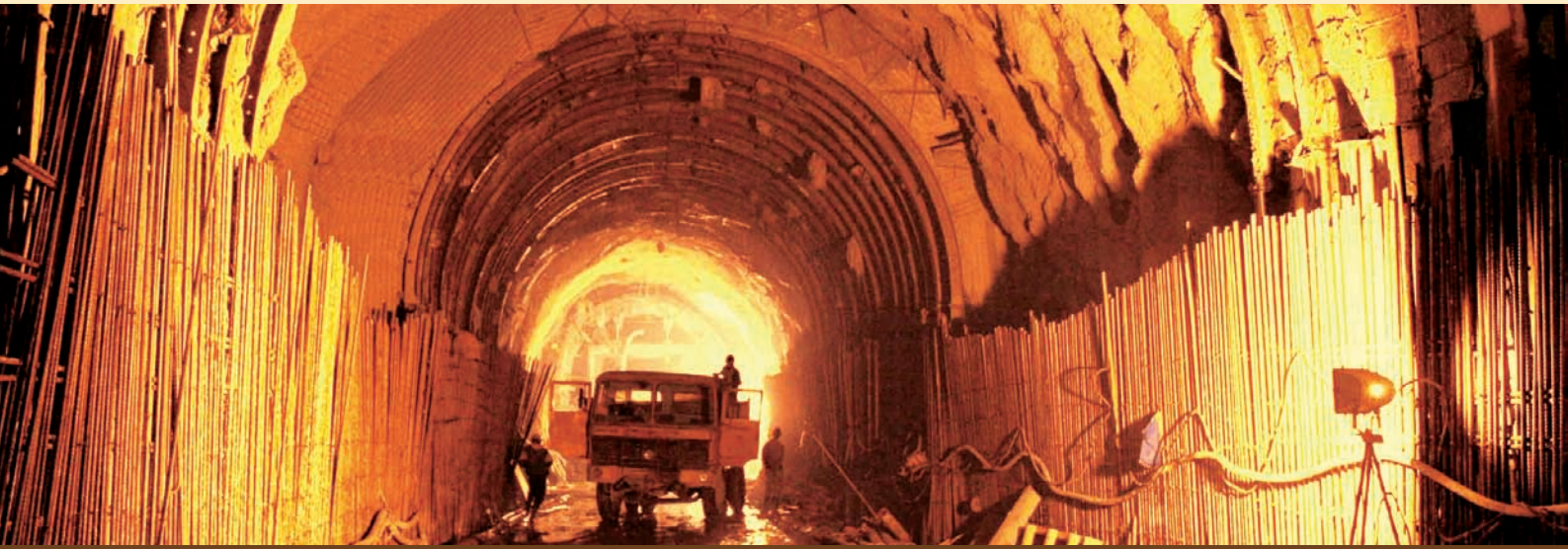
520 MW Parbati-III Project (Himachal Pradesh) - Lining works at Surge Gallery
