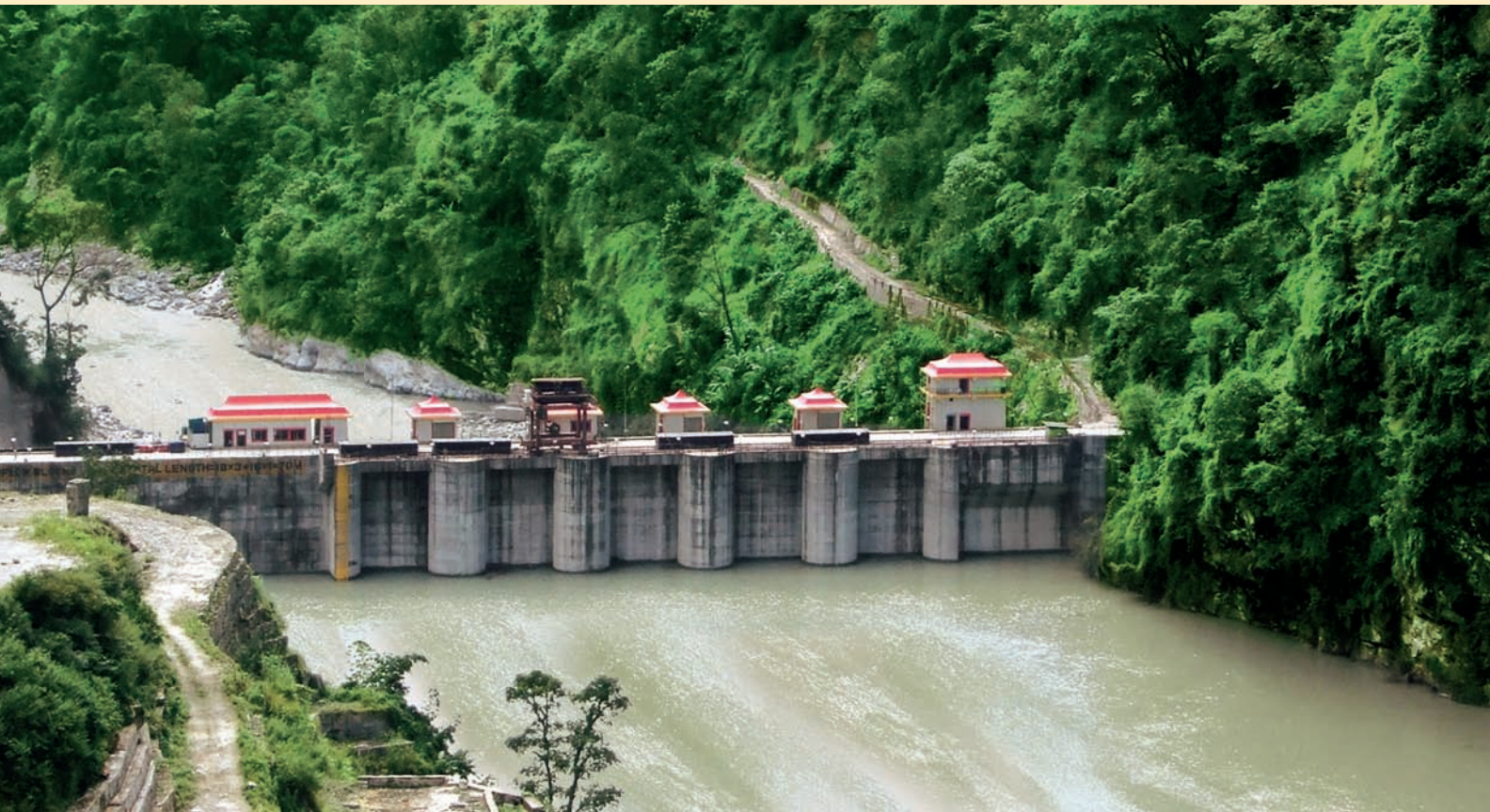
510 MW Teesta-V Power Station (Sikkim) - Upstream view of Dam
