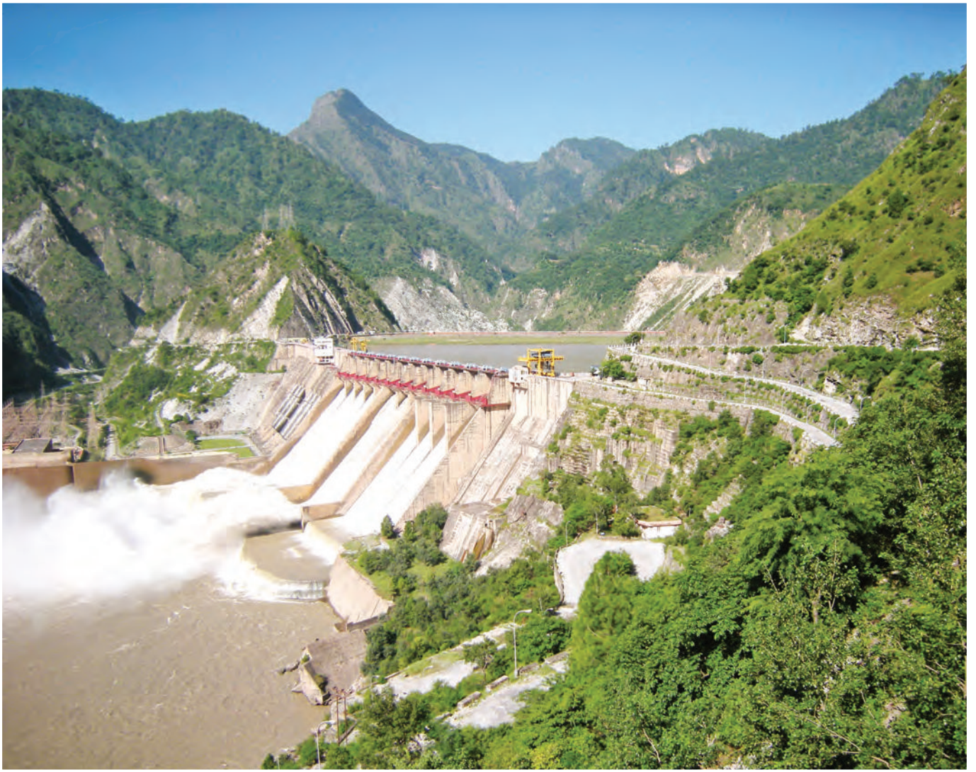
690 MW Salal Power Station (Jammu & Kashmir) - Concrete Dam
