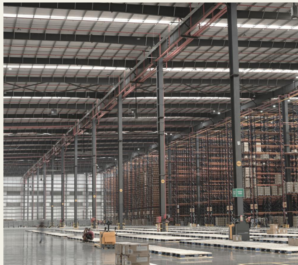
India's largest warehousing box operationalized by Skechers
