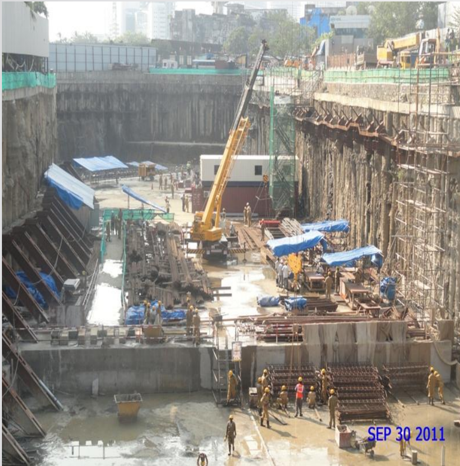
Project Status as on Sep 30, 2011
