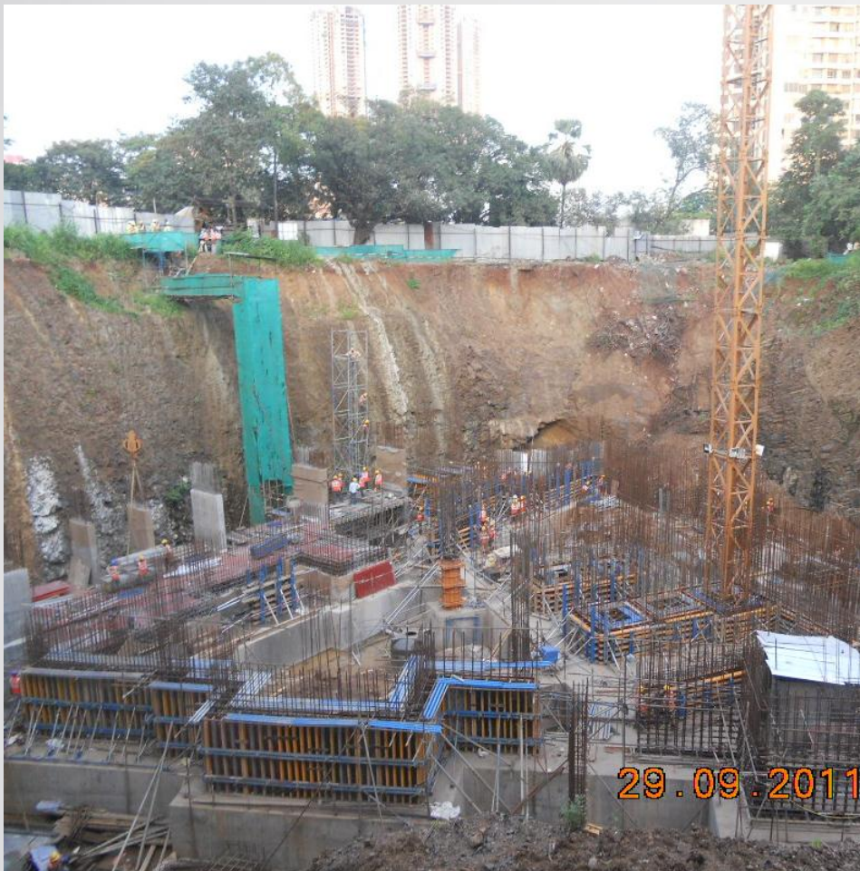
Project Status as on Sep 29, 2011
