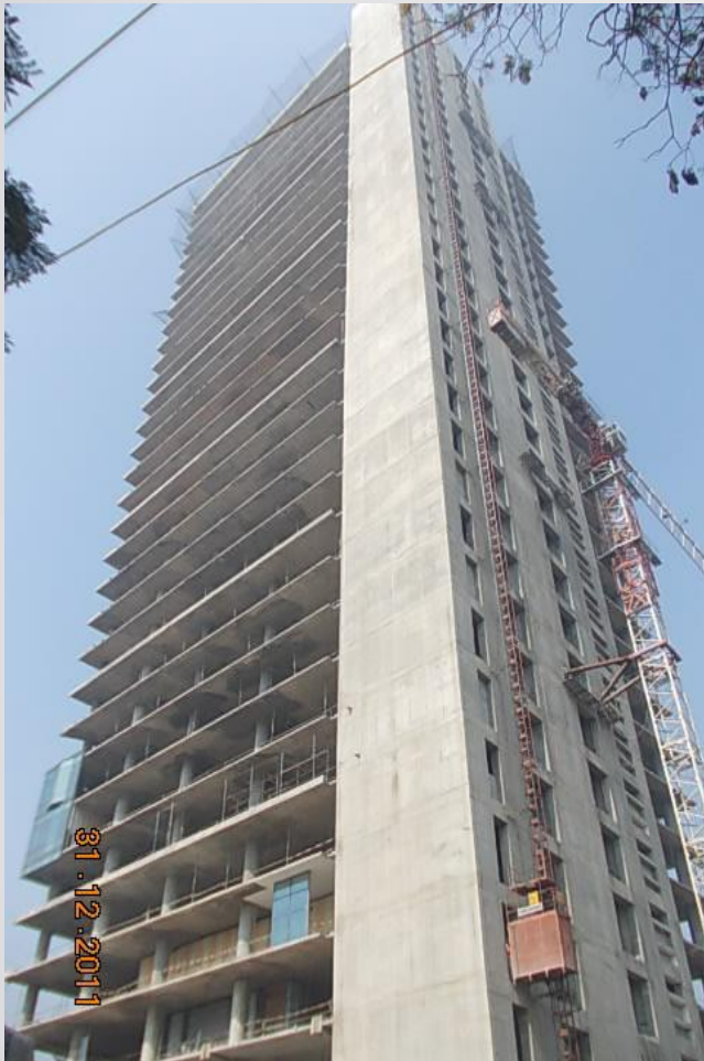
Project Status as on Dec 31, 2011
