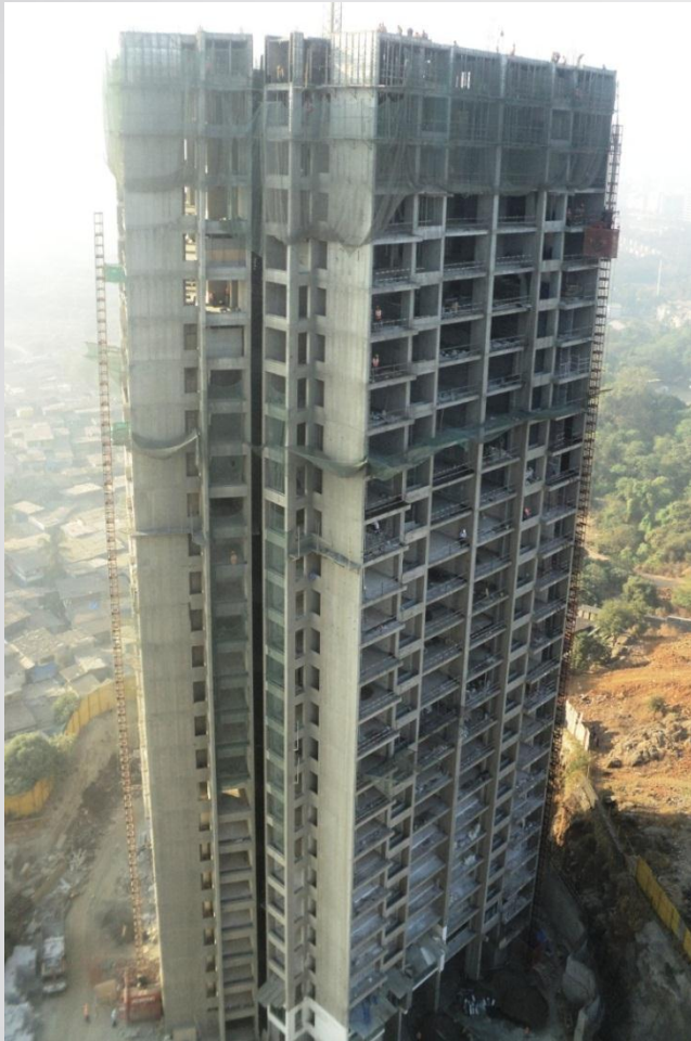
Project Status as on Dec 31, 2011
