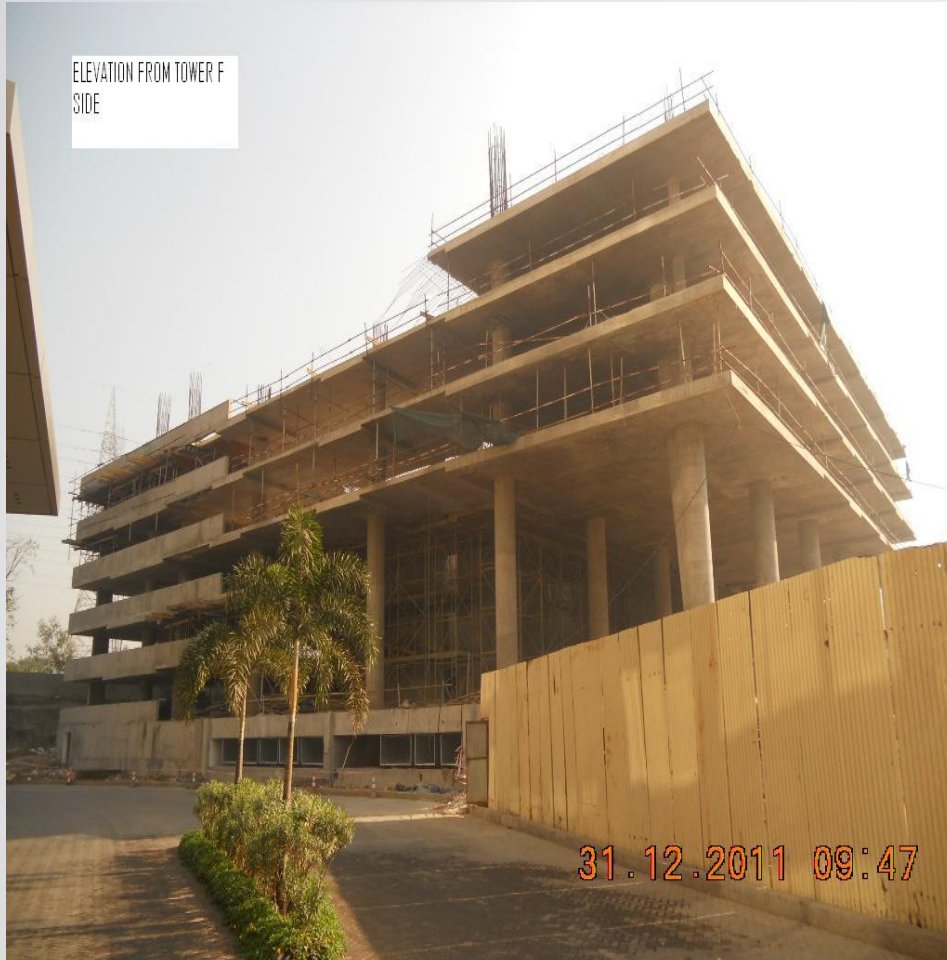
Project Status as on Dec 31, 2011
