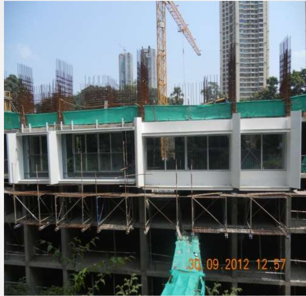
Project Status as on September 30, 2012
