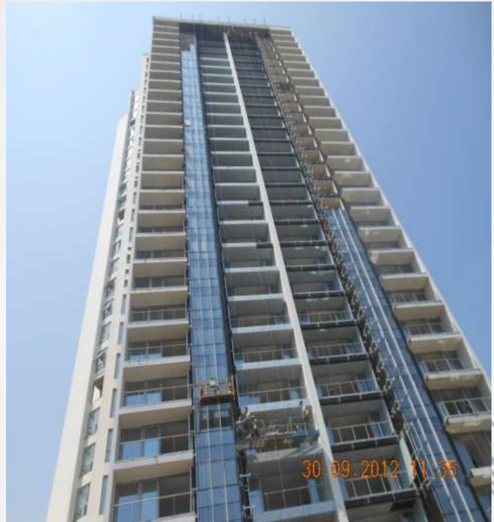
Project Status as on September 30, 2012
