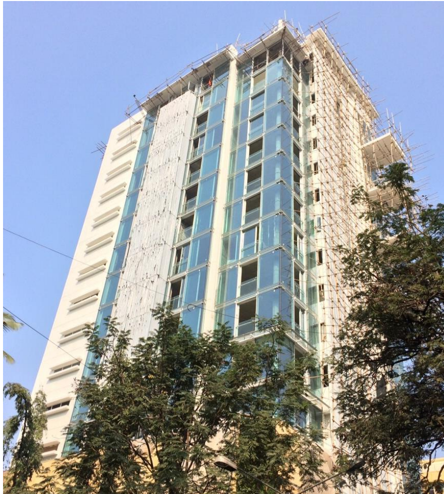
Project Status as on Dec 31, 2014
