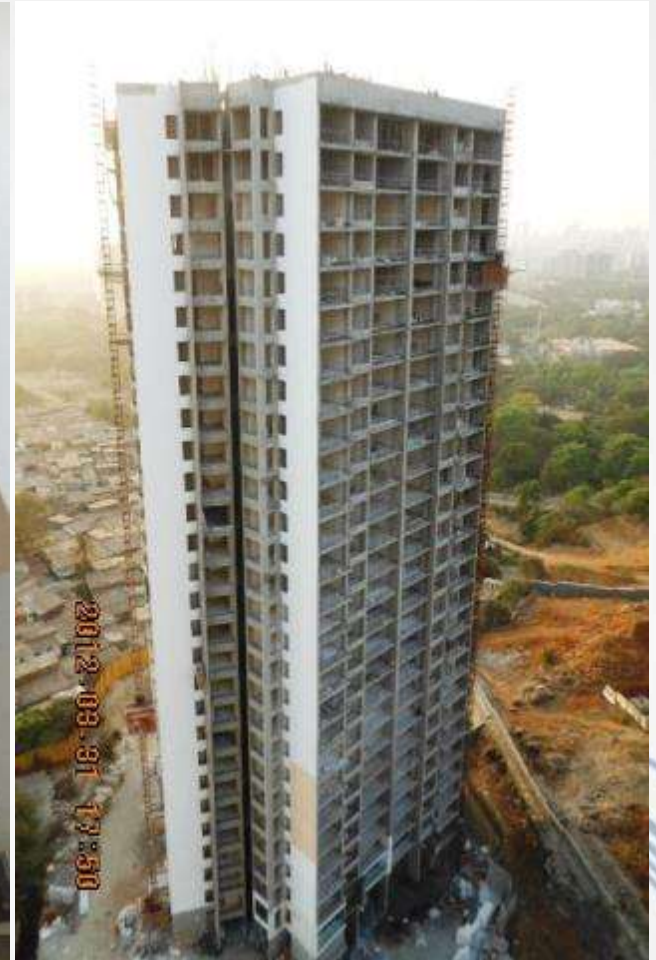
Project Status as on Mar 31, 2012
