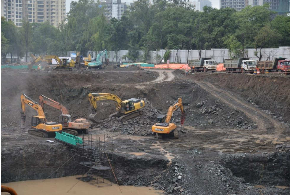
Project status as on Jun 30, 2016
