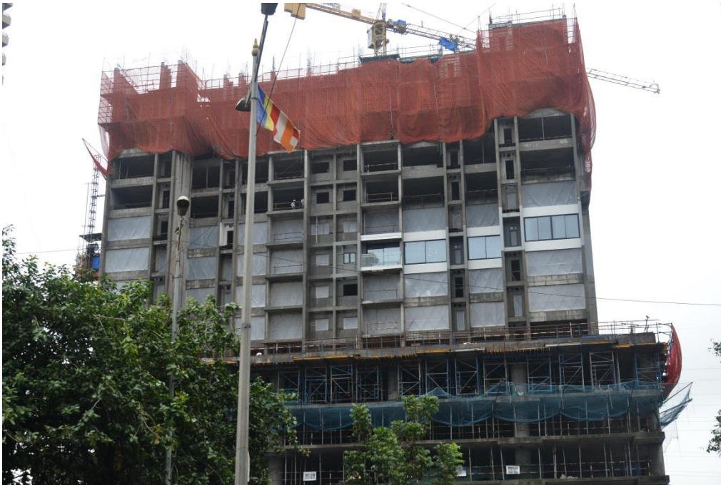
Project Status as on Jun 30, 2016
