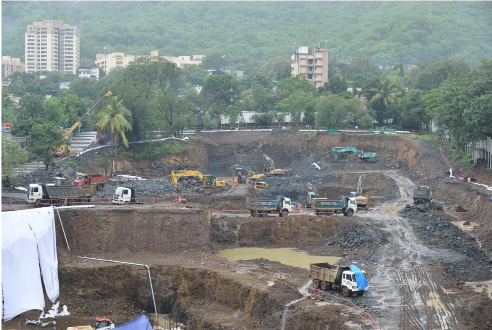
Project status as on Jun 30, 2016
