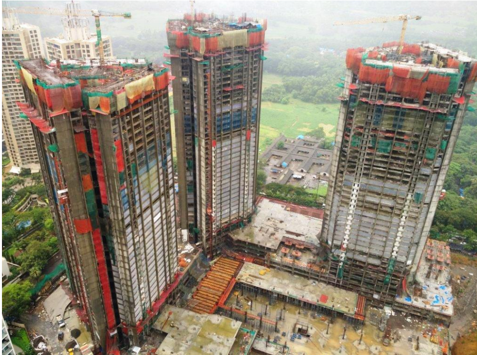
Project Status as on Jun 30, 2016
