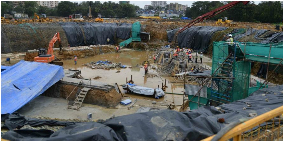
Project status as on Jun 30, 2016
