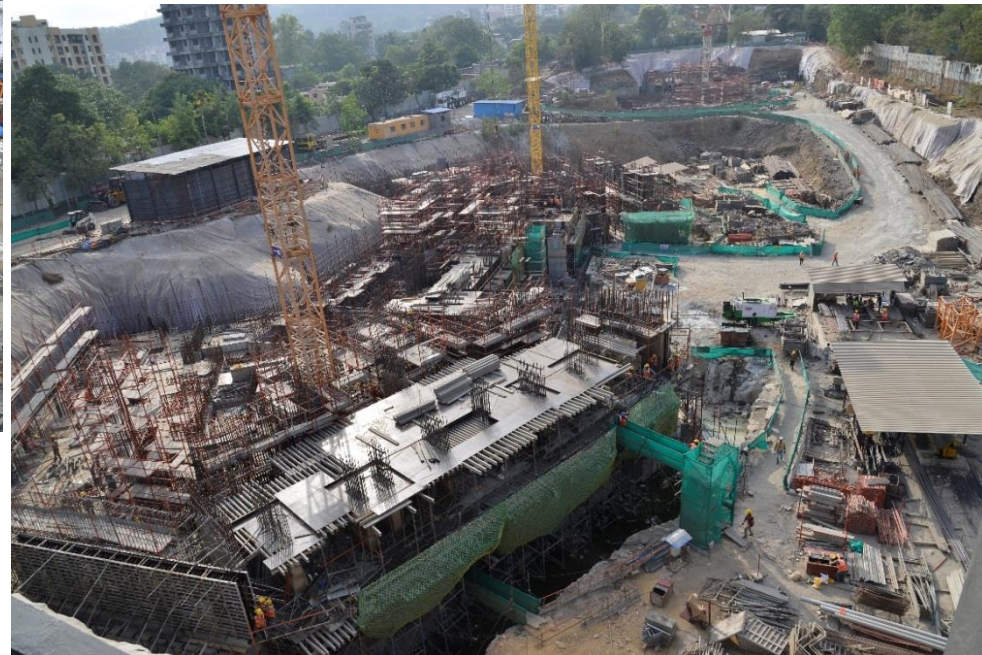
Project status as on Mar 31, 2017
