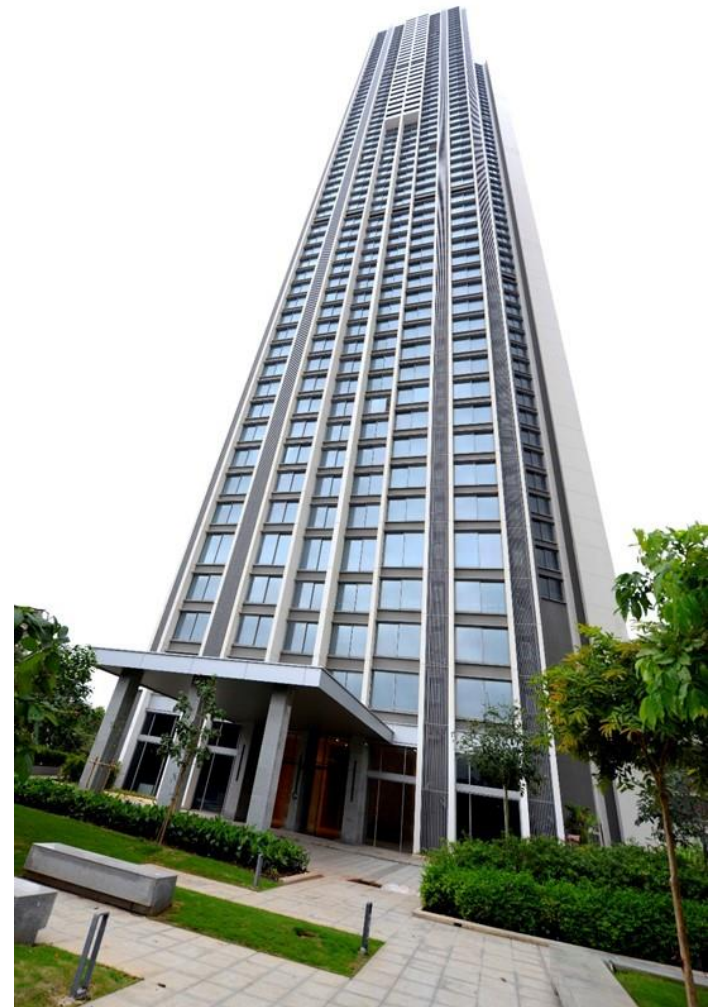
Project status as on Jun 30, 2023
