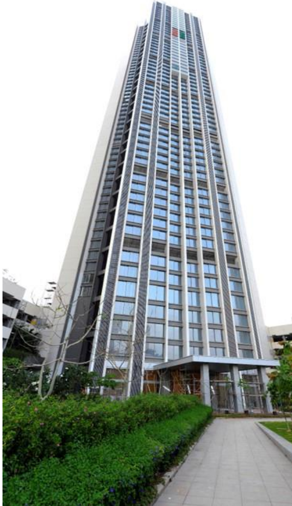
Project status as on Mar 31, 2023
