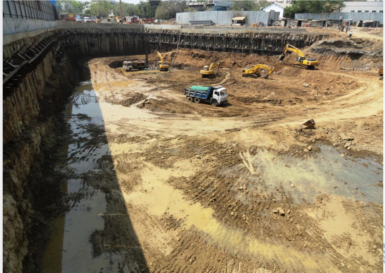
Project Status as on March 31, 2011
