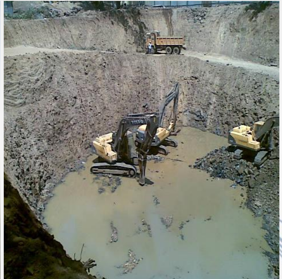
Project Status as on March 31, 2011
