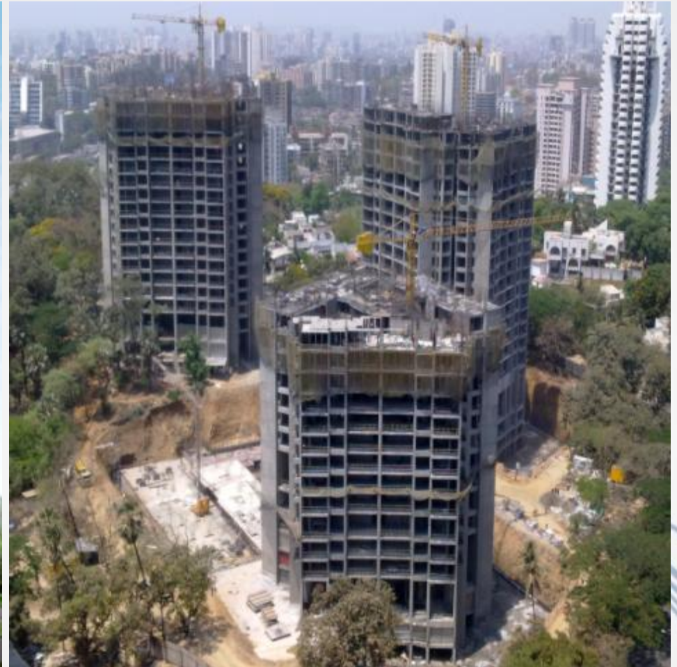
Project Status as on March 31, 2011
