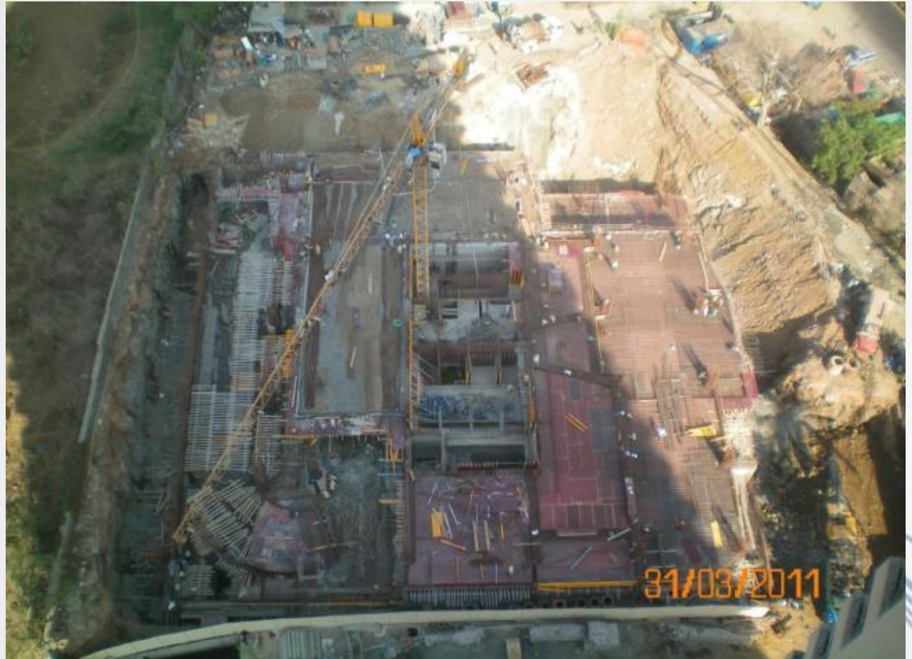
Project Status as on March 31, 2011
