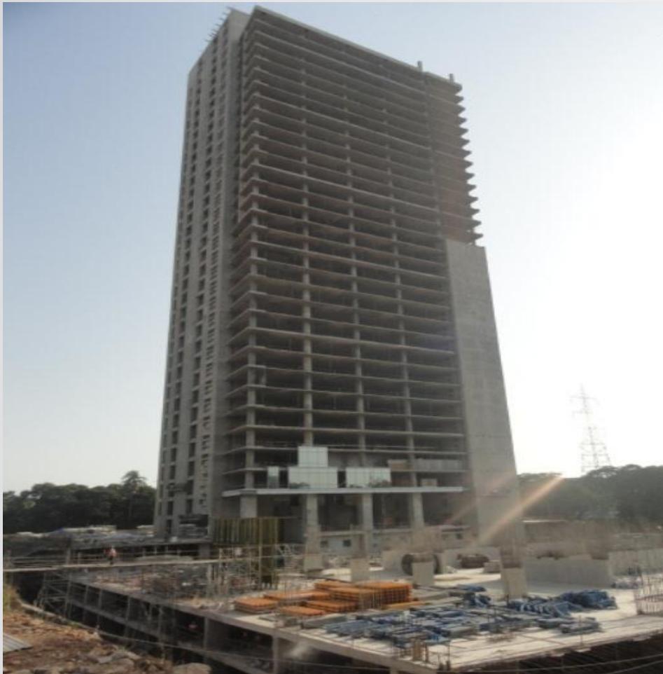
Project Status as on Mar 31, 2012
