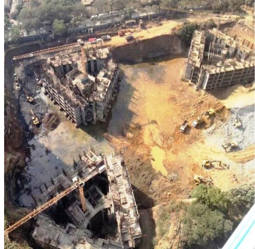
Project Status as on Dec 31, 2013
