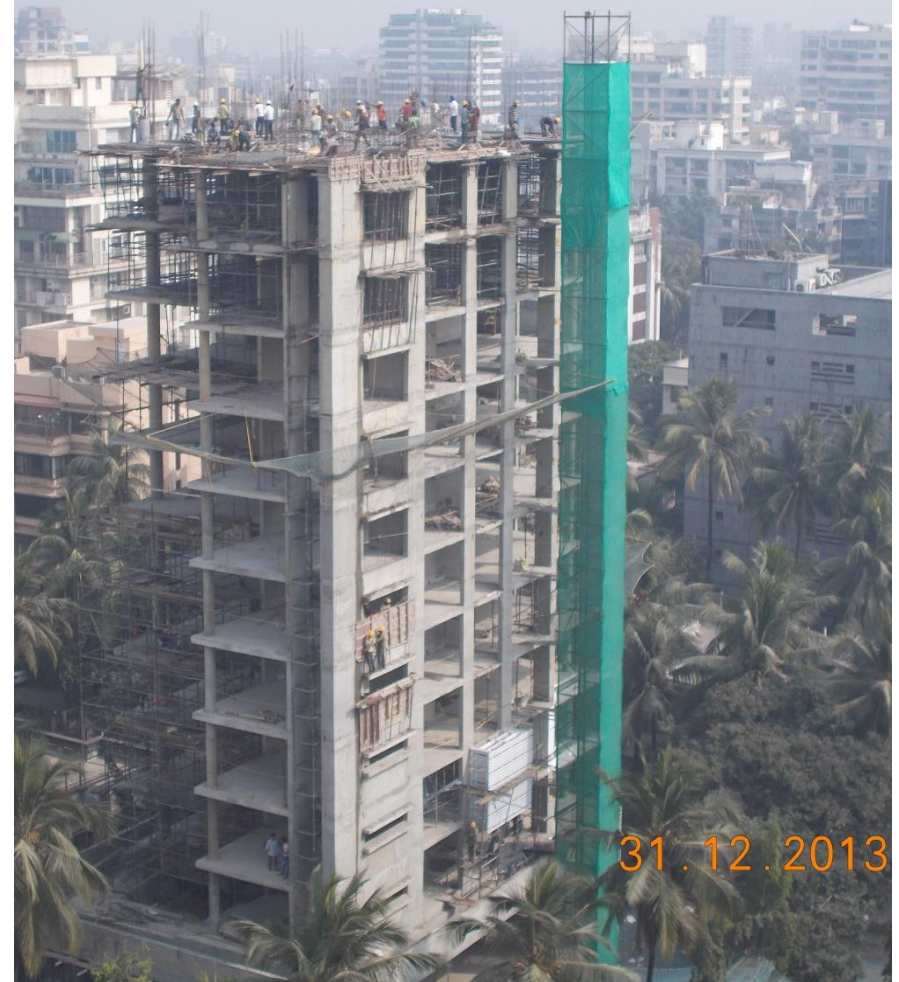
Project Status as on Dec 31, 2013
