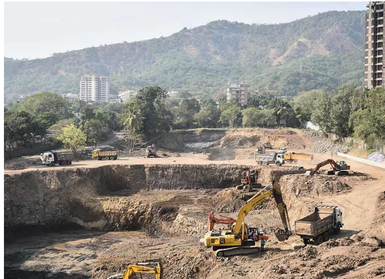
Project status as on December 31, 2015
