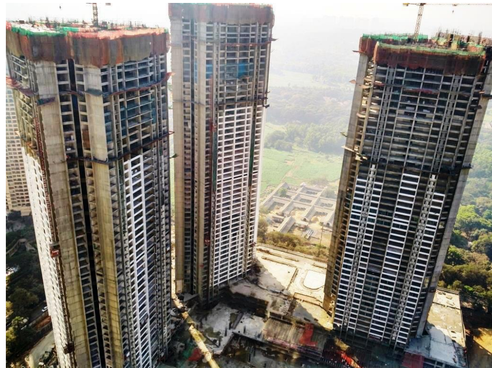
Project Status as on Dec 31, 2016
