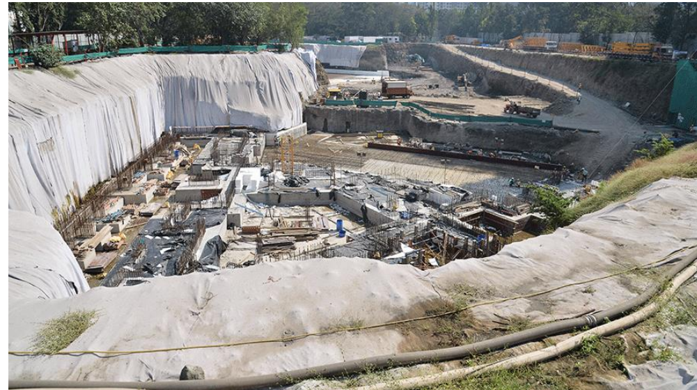
Project status as on Dec 31, 2016
