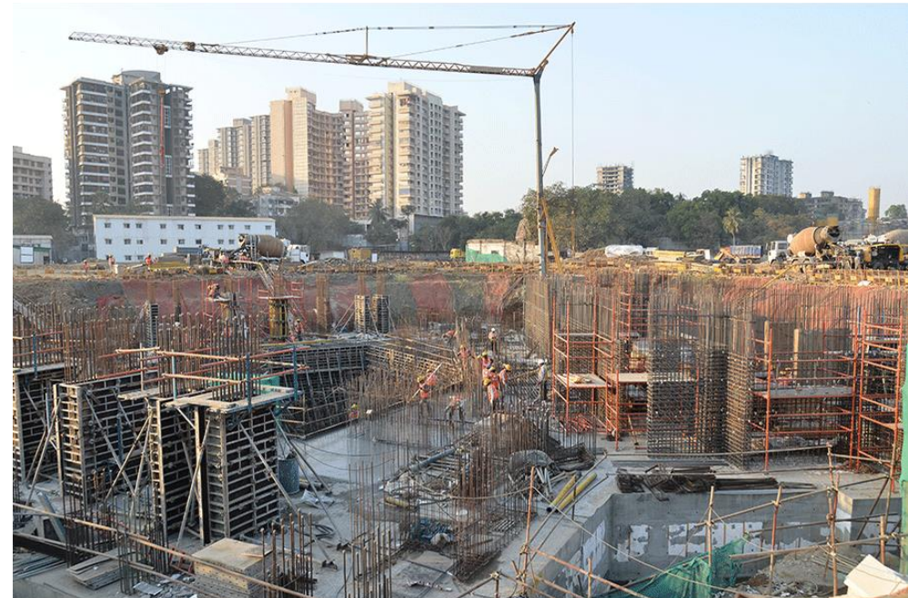
Project status as on Dec 31, 2016
