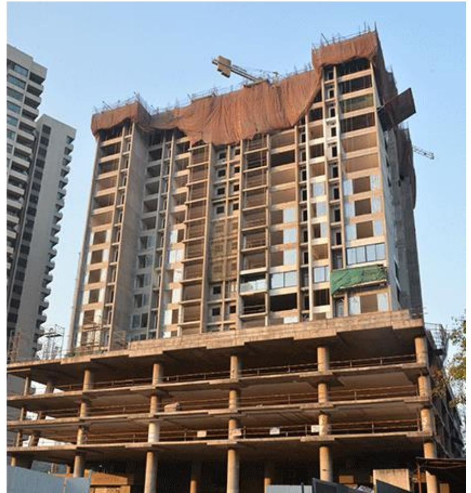
Project Status as on Dec 31, 2016
