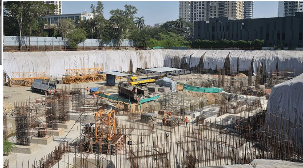
Project status as on Dec 31, 2016
