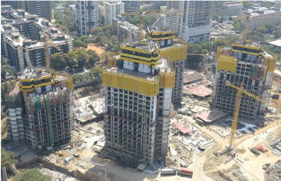
Project status as on Mar 31, 2018
