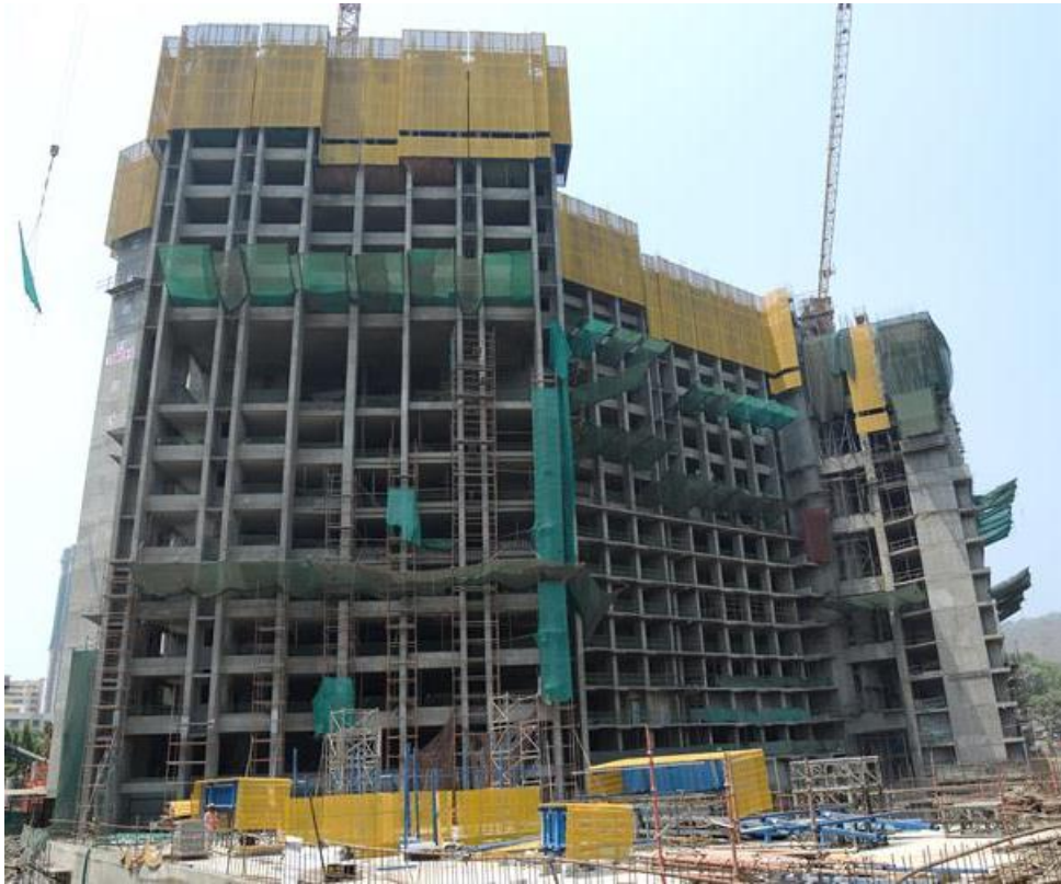
Project status as on Mar 31, 2018
