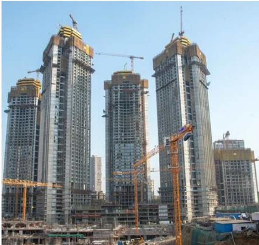
Project status as on Mar 31, 2019
