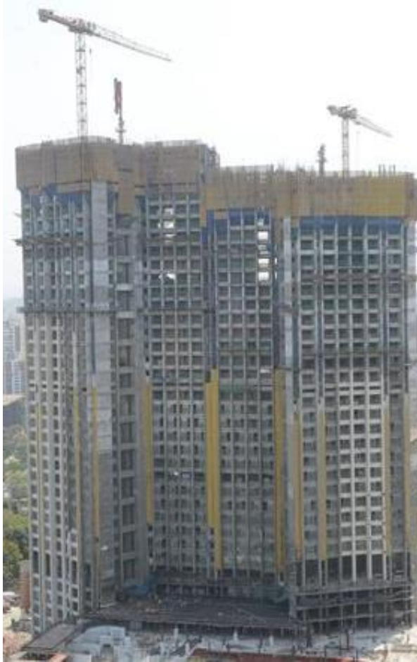
Project status as on Mar 31, 2019
