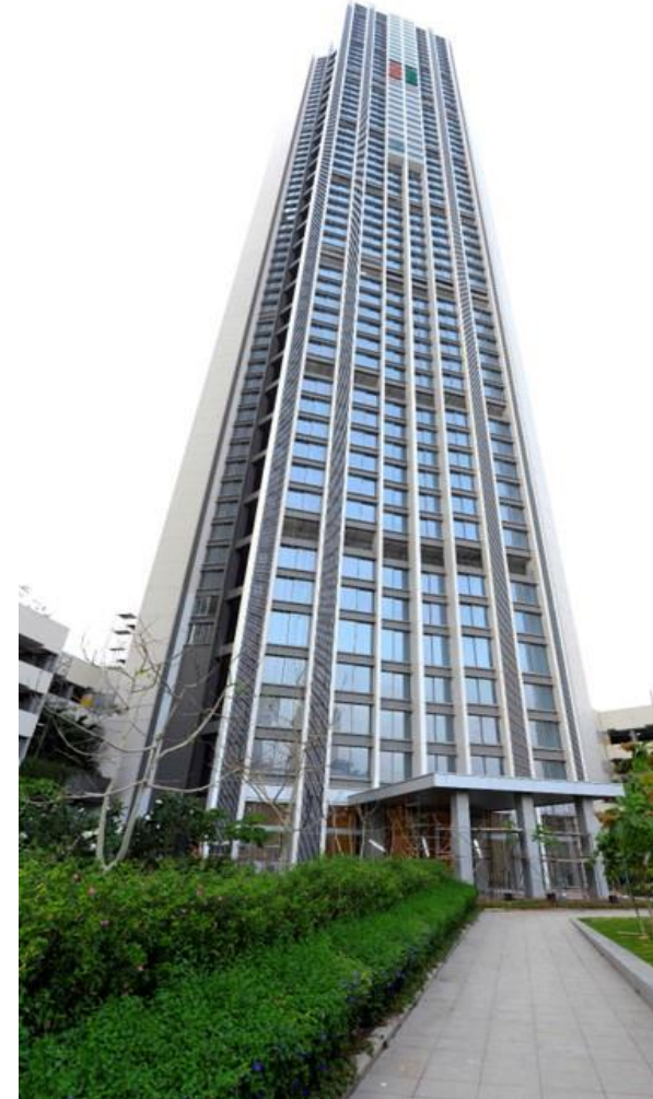
Project status as on Mar 31, 2023
