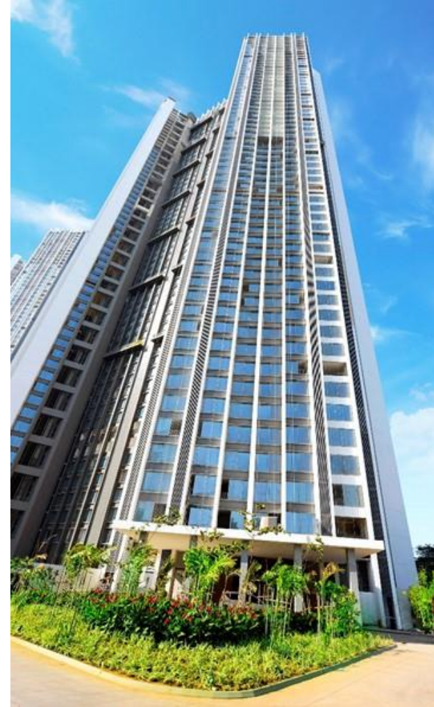
Project status as on Mar 31, 2023
