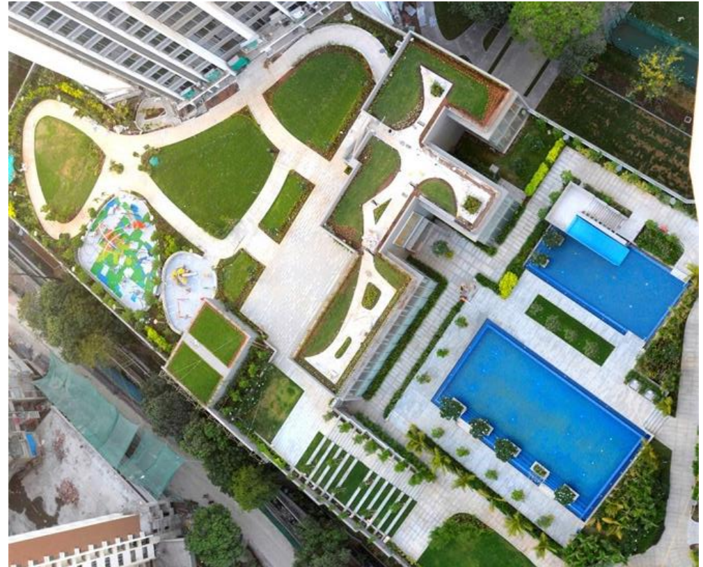
Project status as on Mar 31, 2023
