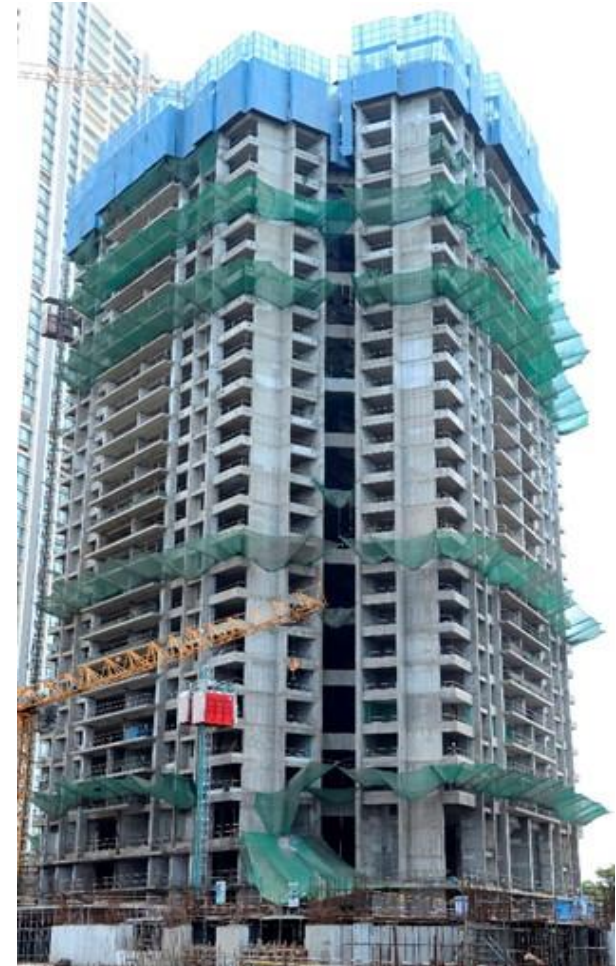
Project status as on Mar 31, 2023
