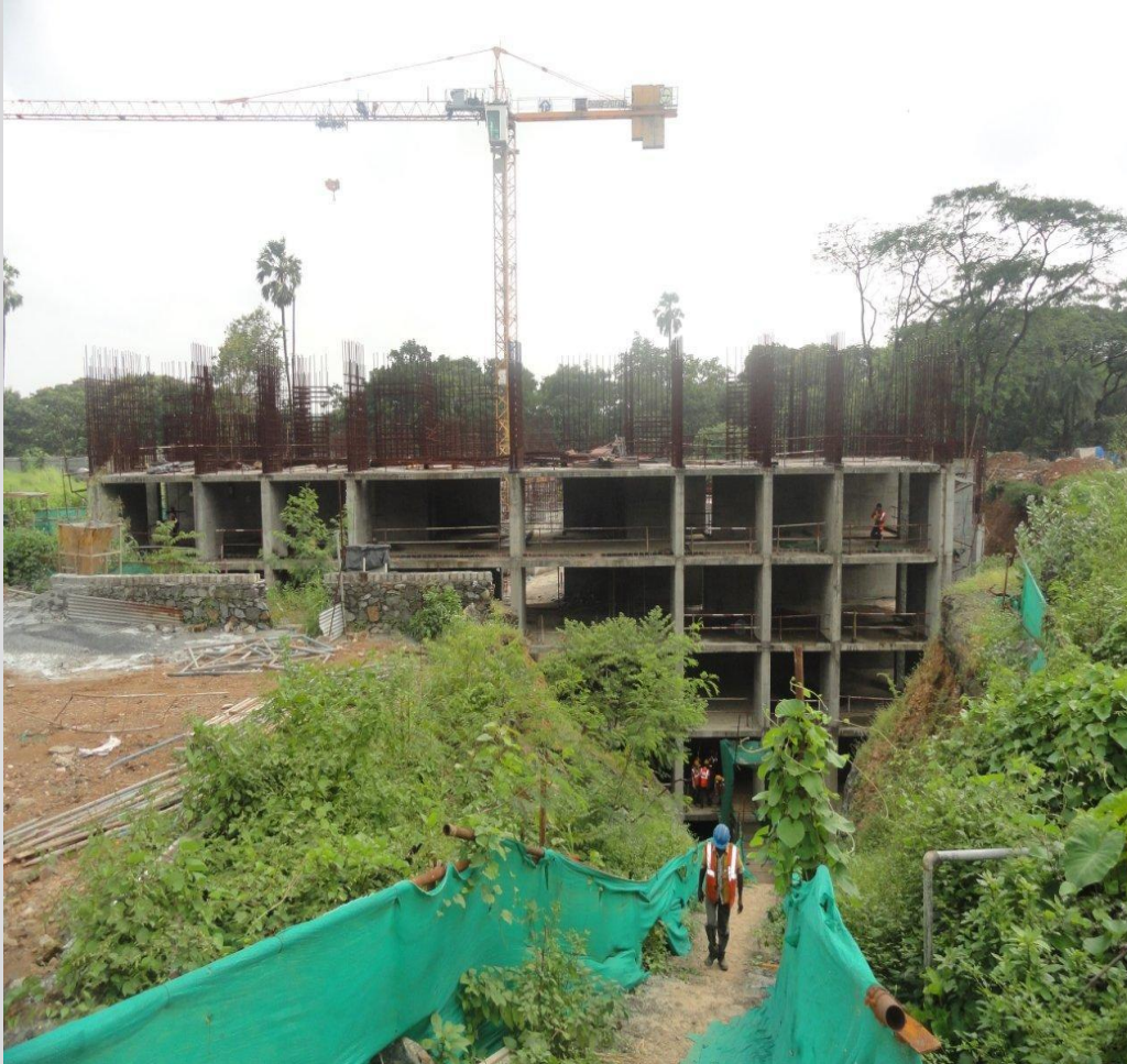
Project Status as on Sep 30, 2013
