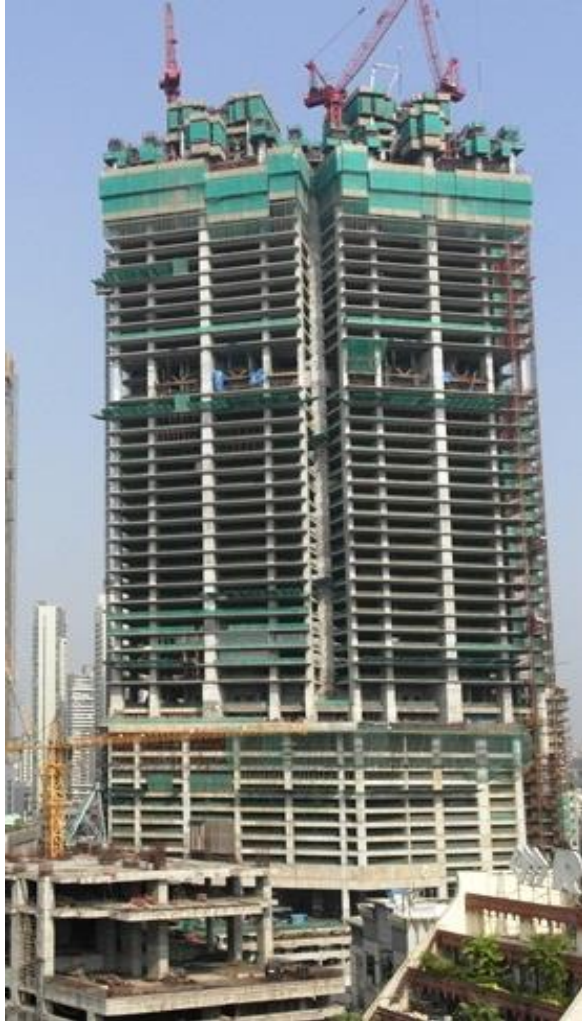
Project Status as on Sep 30, 2014
