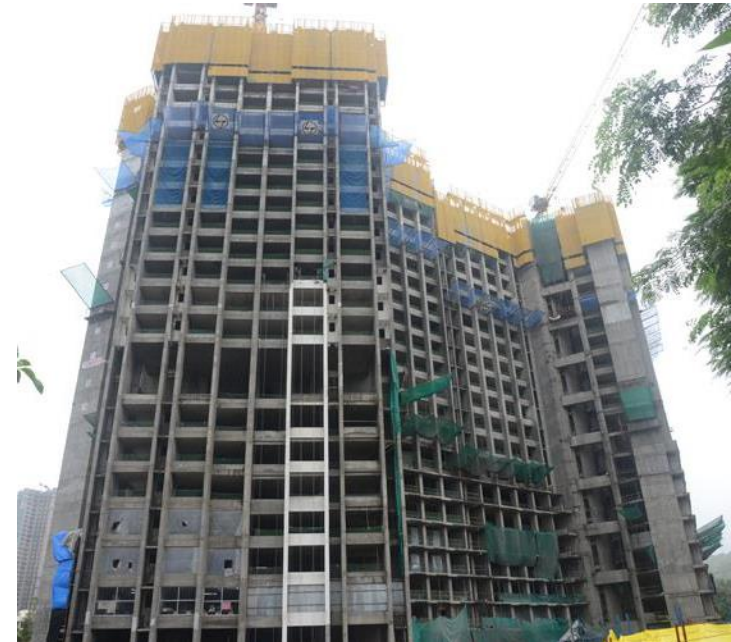
Project status as on Jun 30, 2018
