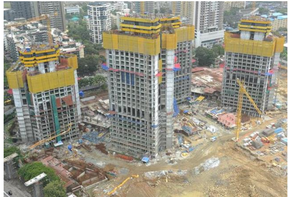
Project status as on Jun 30, 2018
