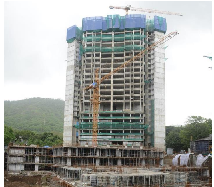
Project status as on Jun 30, 2018
