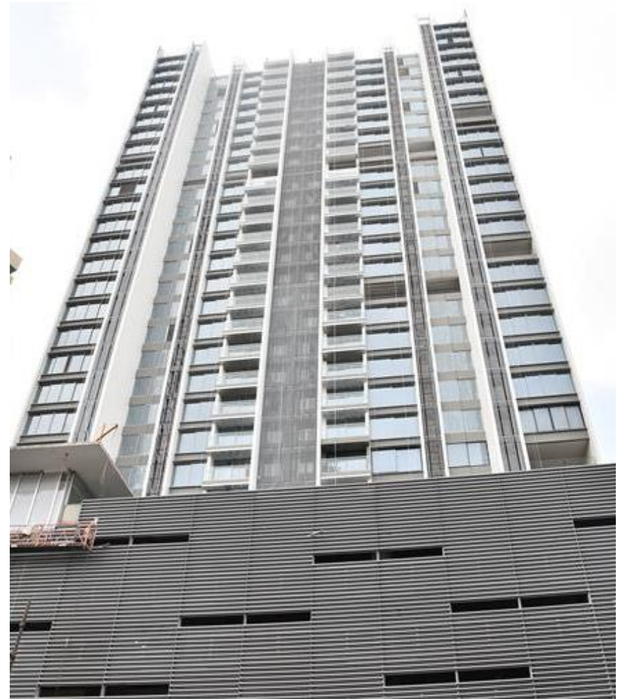
Project Status as on Jun 30, 2018
