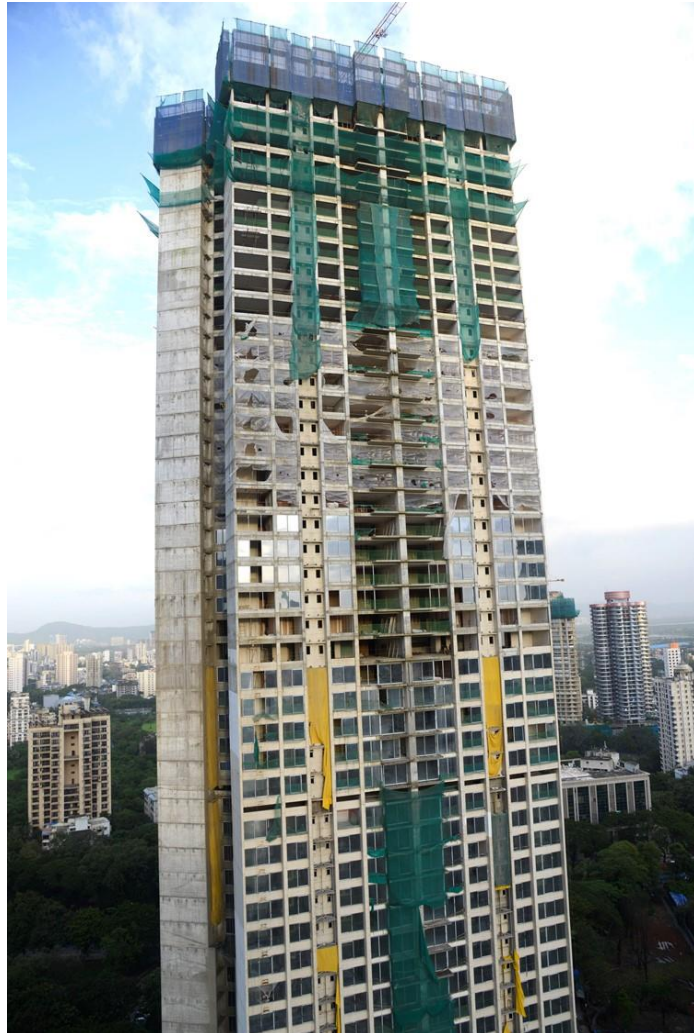
Project status as on Sep 30, 2019
