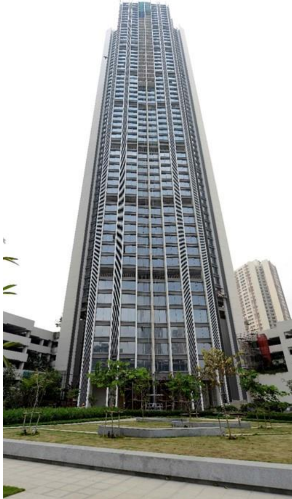
Project status as on Sep 30, 2021
