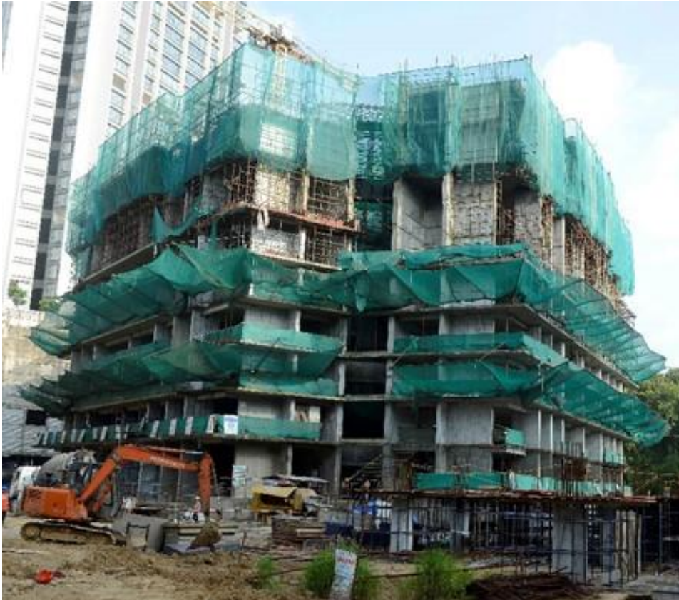
Project status as on Sep 30, 2021
