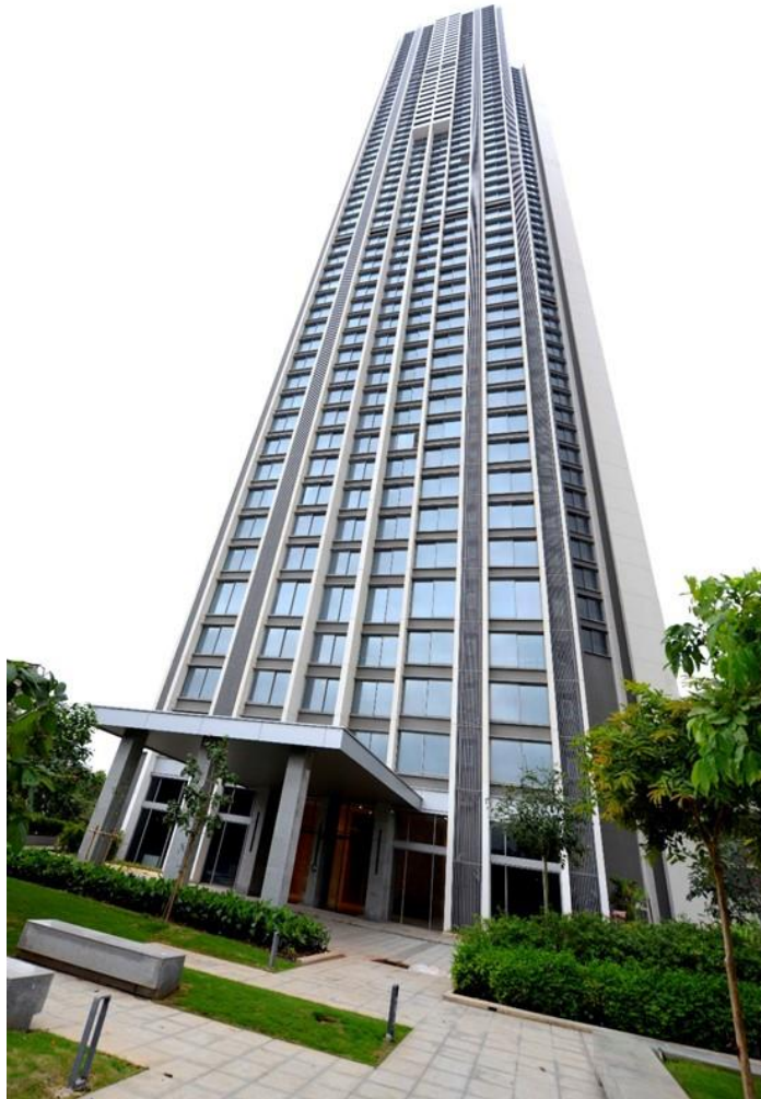
Project status as on Jun 30, 2023
