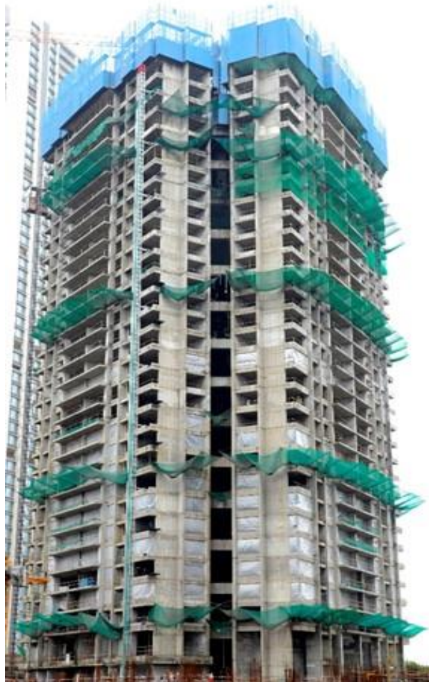
Project status as on Jun 30, 2023
