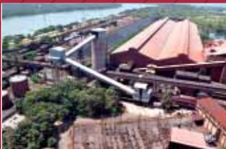
View of Pellet Plant
