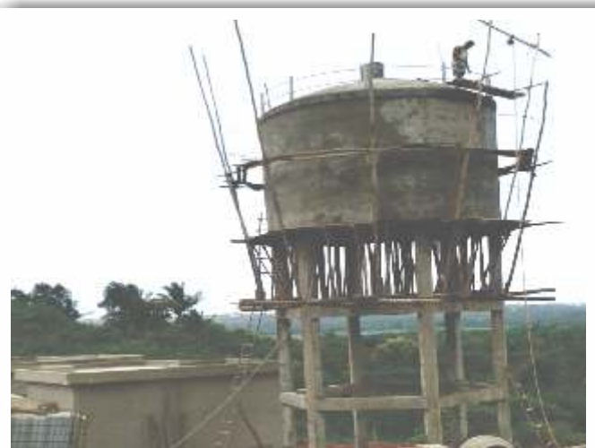
50000 Ltrs capacity water tank under construction by KIOCL for the resettlement Colony at Porkodi
