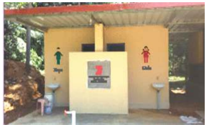
Toilets constructed under 'Swachh Bharat-Swachh Vidyalaya Abhiyan' at Sri Mujilnaya Aided Higher Primary School, Nooralbettu
