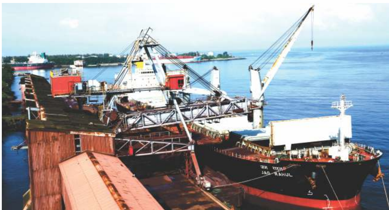
Ship Loading Facility at Pellet Plant, Mangalore
