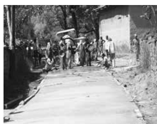
RCC road construction in village
