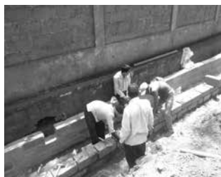
Drain construction in Siltara
