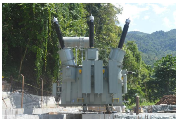
10MVA STATION TRANSFORMER ERECTION COMPLETED
