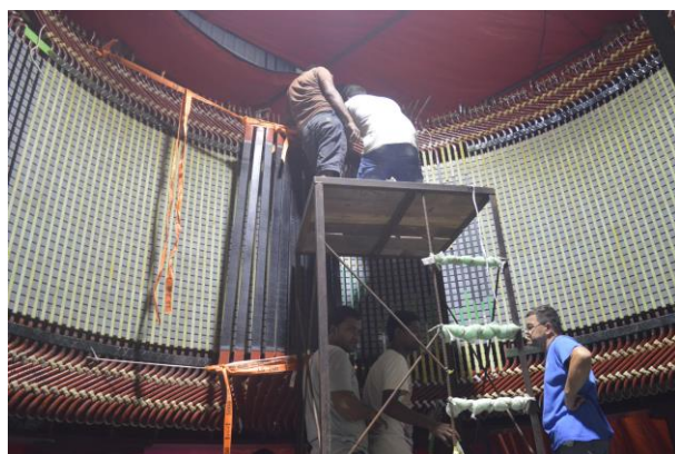
UNIT-2 STATOR WINDING UNDER PROGRESS
