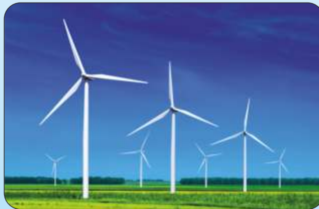
47.6 MW - KWPS (Wind Field)
