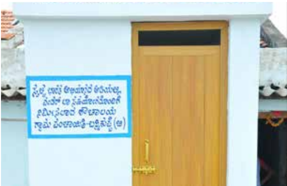
To uplift health and sanitation in rural areas the company has constructed 87 individual toilets (11 in FY 2017-18) in villages under Swachh Bharat mission.
