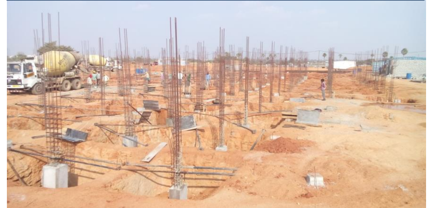
CONSTRUCTION OF ENTRANCE BUILDING
