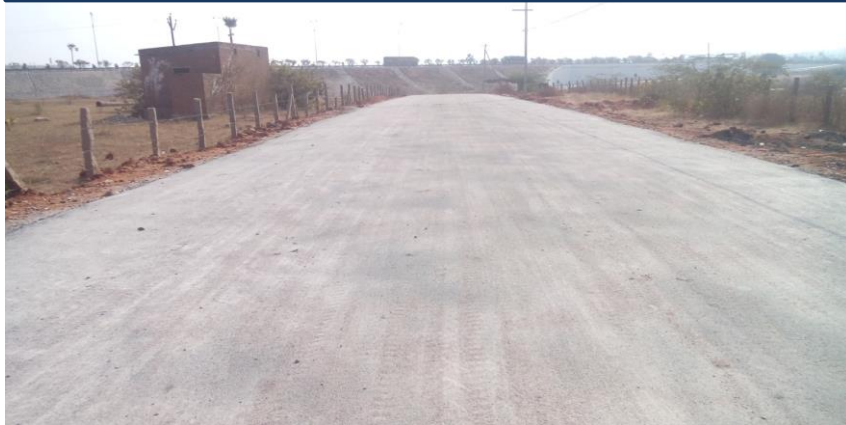
CONSTRUCTION OF APPROACH ROAD
