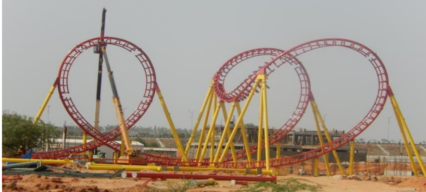
CONSTRUCTION OF ROLLER COASTER
