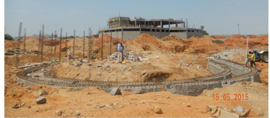
CONSTRUCTION OF WONDER SPLASH
