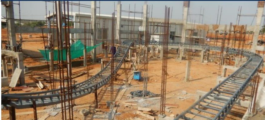
CONSTRUCTION OF TERMITE COASTER TRACK
