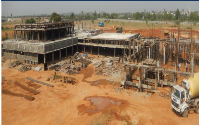
CONSTRUCTION OF ENTRANCE BUILDING
