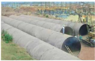
3750 mm dia M.S.pipes with coal-tar coating under erection at D.B. Power plant near Raigarh in Chhattisgarh State for cooling water supply pipe line system.
