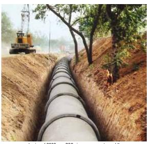
Laying of 2000 mm PSC pipes on concrete craddle bedding at Ghaziabad water supply project
