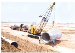
Laying of 2000 mm dia PSC pipes at Pulikanuma Lift Irrigation Scheme in A.P.
