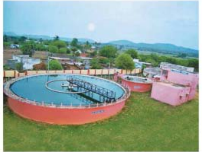
Water Treatment Plant
