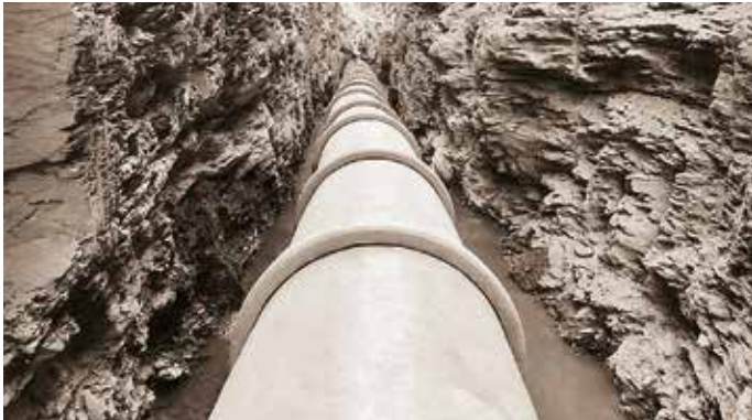
4.05 km, 1800 mm dia PSC pipes for Morjampadu Lift Irrigation Scheme
