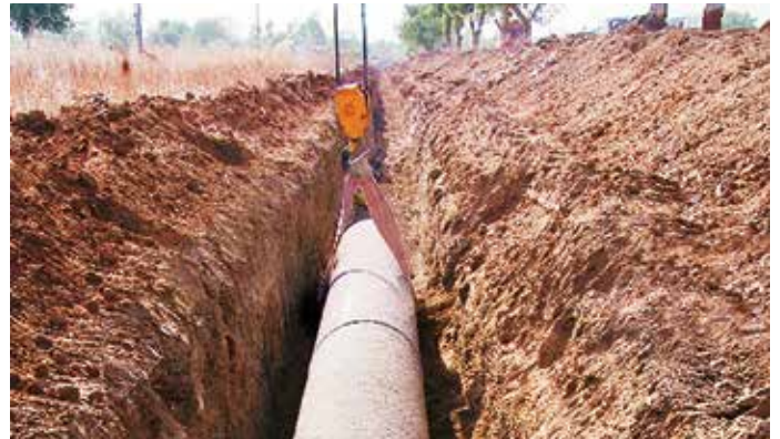
33.39 km, 800 mm dia BWSC Pipes for Chalisgaon Water Supply Scheme
