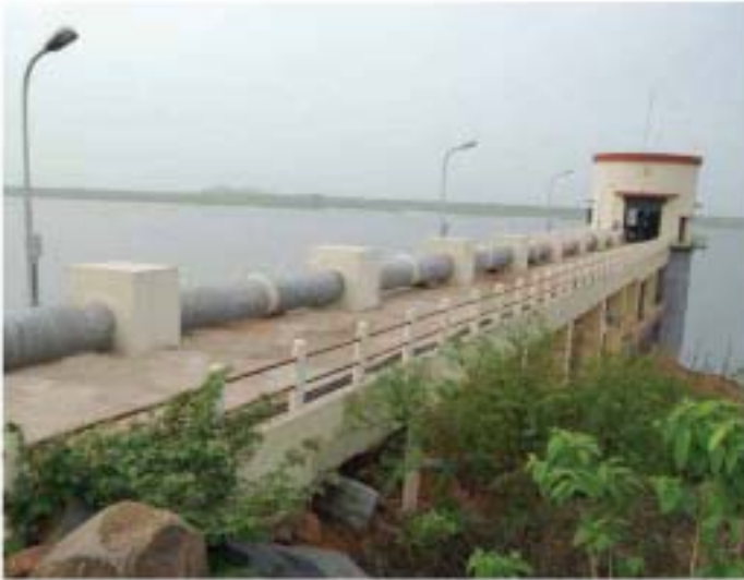
Intake Well cum Pump House
