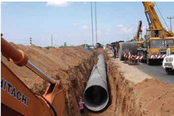
2200 mm dia MS Pipes for Krishna Drinking Water Supply Project Phase-III Package-IV, Andhra Pradesh
