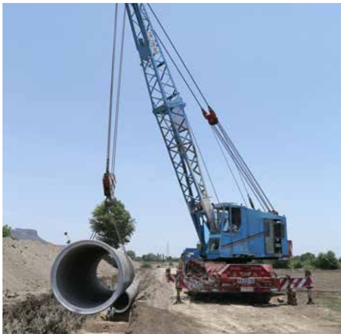
1500 mm dia PCC Pipes for Chilhwadi Pipeline Project, Maharashtra
