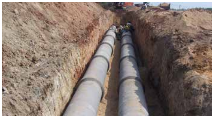
900 mm dia PSC pipeline laying for IFFCO Kisan SEZ Nellore, Andhra Pradesh
