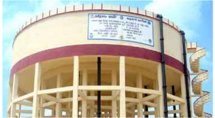
15 Lakh Liter capacity Elevated Storage Reservoir for Palladam Water Supply Project, Tamilnadu
