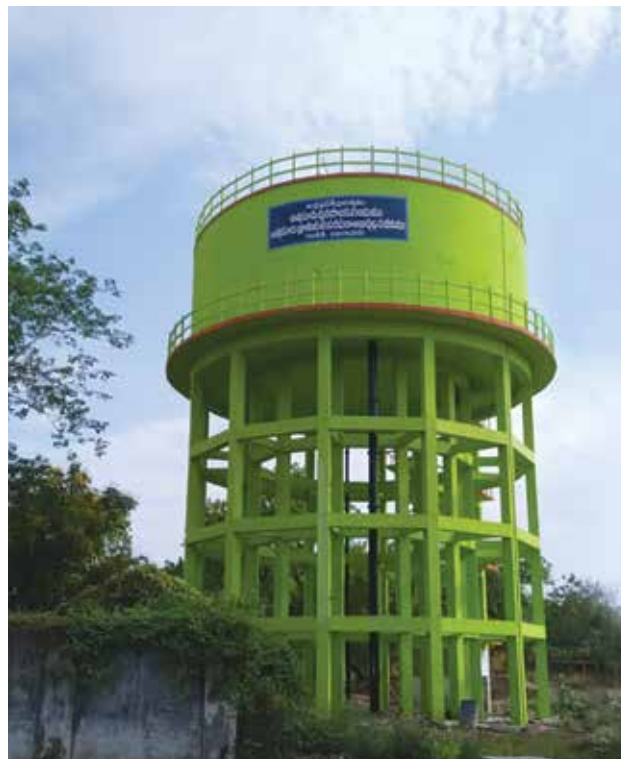
7 Lakh litre capacity Elevated Storage Reservoir for Atmakur Project, Andhra Pradesh
