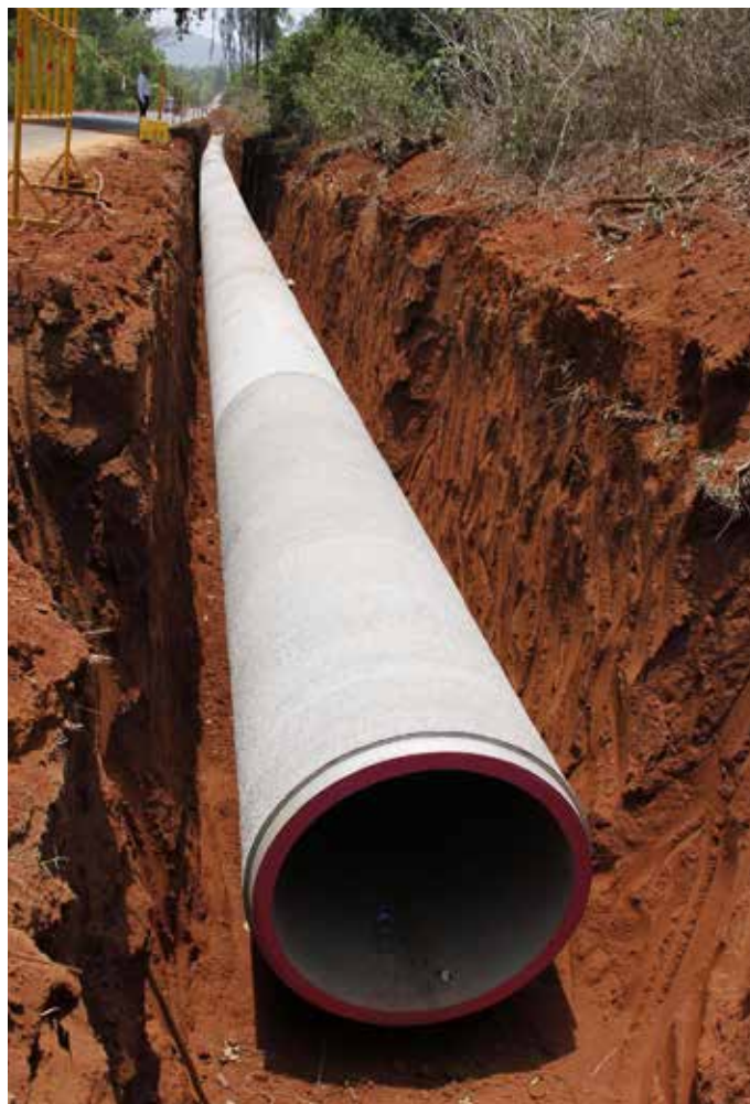
1200 mm dia PCC pipes laying for Tillari Water Supply Scheme, Maharashtra
