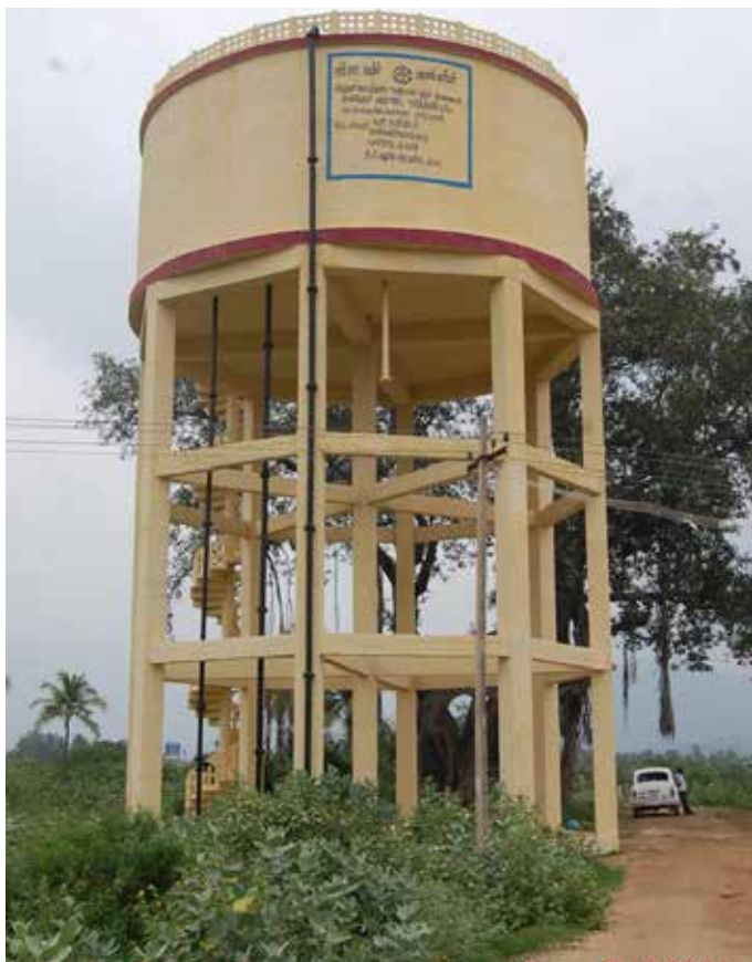
3 Lakh litre capacity Elevated Storage Reservoir at Rajapalayam Project of TWAD Board, Tamilnadu
