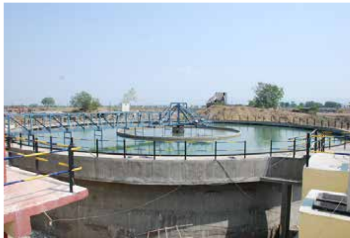
26 MLD Water treatment plant at Chalisgaon City Water Supply Scheme, Maharashtra
