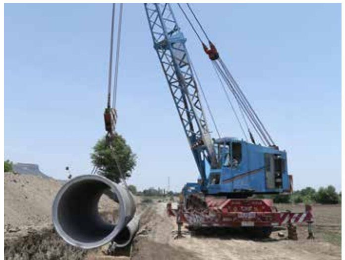
1500 mm dia PCC pipes laying for Chilhwadi Pipeline project, Maharashtra
