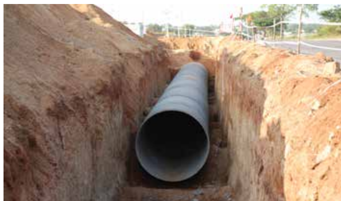
2200 mm dia MS pipeline for Krishna Drinking Water Supply Project Package-IV Phase-III, Telangana
