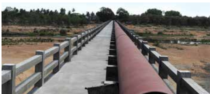
360 Mtrs length foot bridge at River Kollidam for 700 mm dia MS Pipeline at CWSS to Pudukottai, Tamilnadu
