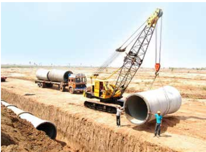
2000 mm dia PSC pipeline laying for Pulikanuma LIS in Kurnool District in Andhra Pradesh
