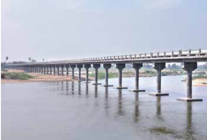
580 meters long Foot Bridge at Cauvery River carrying 711 mm dia M.S. Pipeline for CWSS to Pudukottai in Tamilnadu.
