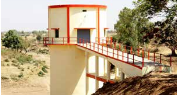
Intake Well for Guna Water Supply Projects in Madhya Pradesh
