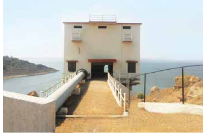
RCC Jackwell 10 meters dia in Girna Dam for Chalisgaon Water Supply Scheme in Maharashtra
