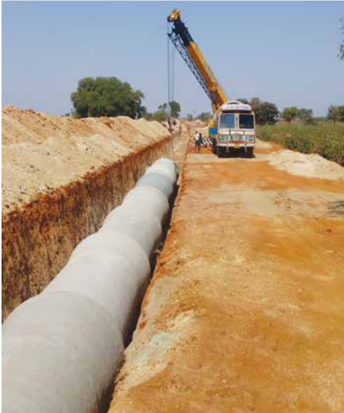
1900 mm dia PSC pipeline laying at Pulakurthy LIS in Kurnool District in Andhra Pradesh
