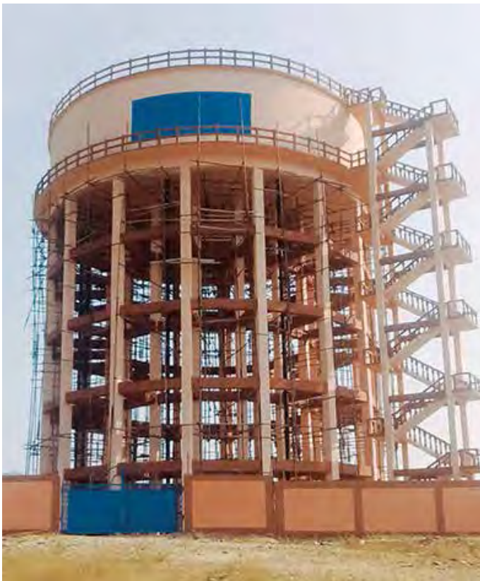
1000 KL OHBR at Maruthomma Nagar for Badvel Project in Andhra Pradesh
