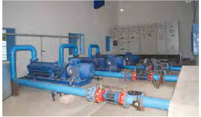
12 x 6 Mtr Pump House at Morthad for Balkonda Project in Telangana
