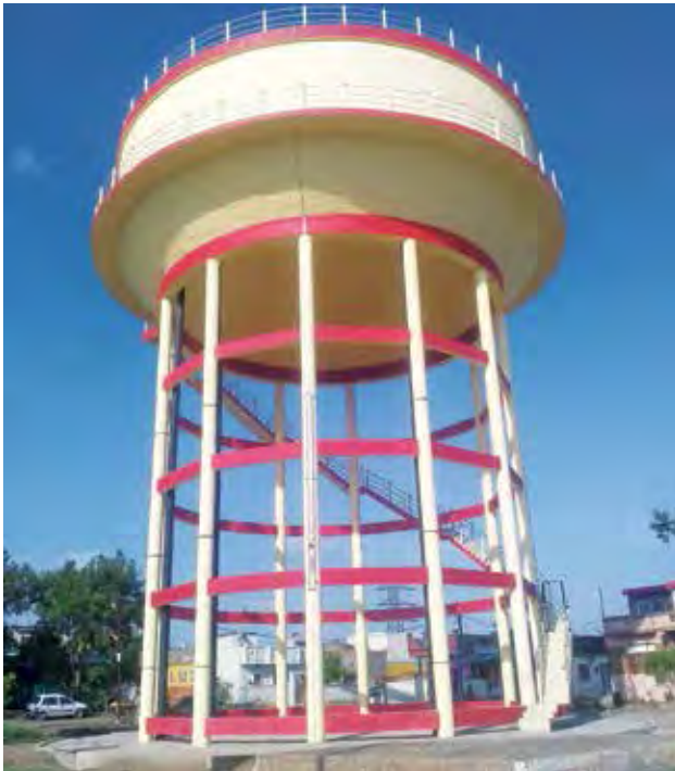
1500 KL capacity OHT at Uttam Nagar for Dewas Water Supply Scheme, in Madhya Pradesh
