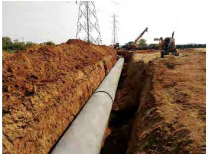
1200 mm dia MS pipeline laying at Jurala Project in Telangana
