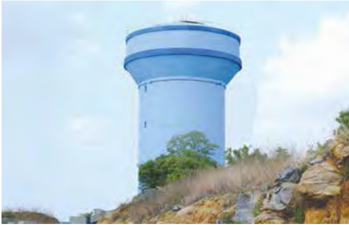
400 KL x 15mtr staging OHBR at Balkonda Hill for SRSP-Balkonda Project in Telangana
