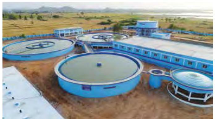
Water Treatment Plant for Jurala Project, in Telangana
