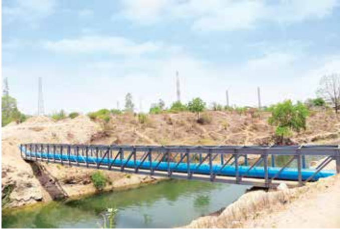
Durry Canal Trussbridge with 700 MM dia MS pipeline for Korba Water Supply Scheme, in Chhattisgarh
