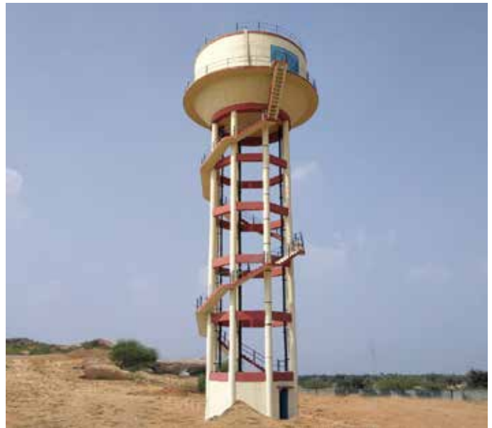
300 KL x 24 mtr. staging OHBR at Jahazpur Project, in Rajasthan
