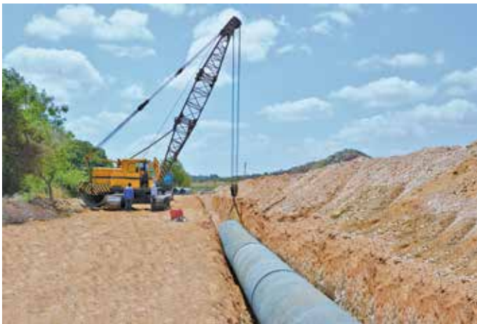
1600 mm dia Prestressed Concrete Cylindrical Pipes laying & jointing at Karnataka Power Corporation Ltd, Bellary Project, in Karnataka.
