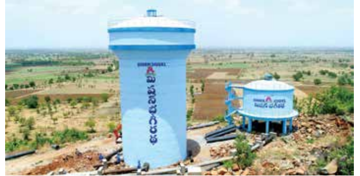
300 KL OHBR & 150 KL GLBR at Argul for Balkonda (TDWSP) Project, in Telangana.
