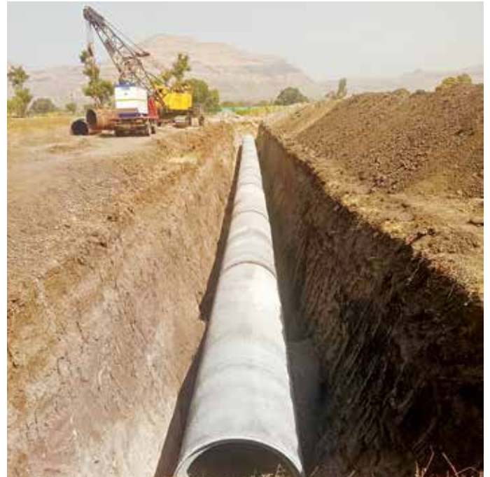
1300 MM dia PCCP pipeline laying for Chilhwadi Pipeline Project, in Maharashtra
