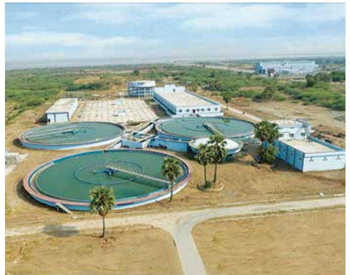
160 MLD Water Treatment Plant at Murrur village, Yellampally, Peddapali, Ramagundam for TDWSP Circle, Karimnaagr, in Telangana.
