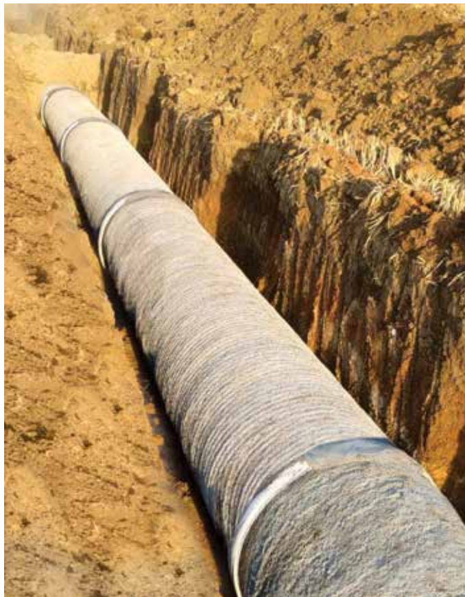
700 mm dia PCCP Pipeline laying at Pauni Lift Irrigation Scheme, in Maharashtra
