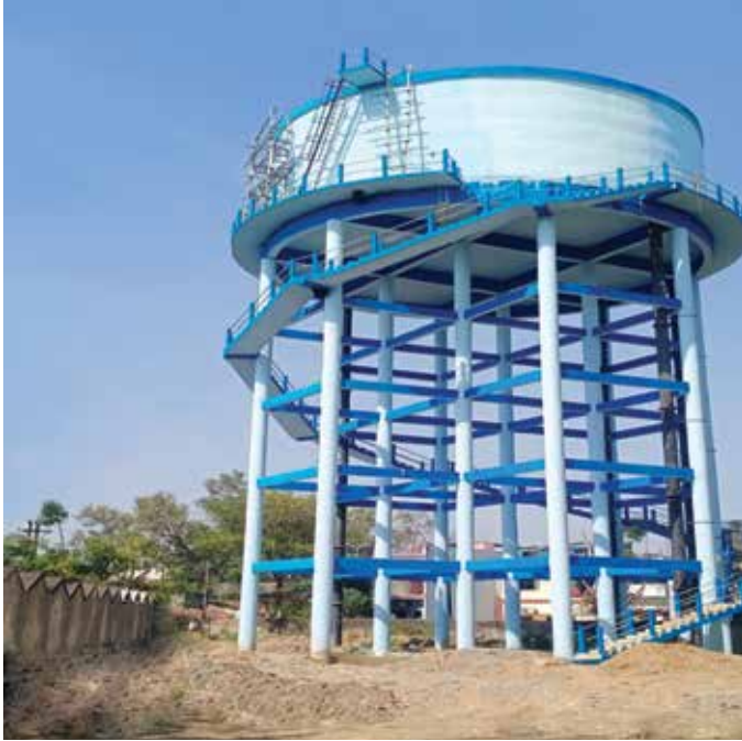
880 KL Overhead Tank staging 21 Mtr at Torwa for Bilaspur Water Supply Scheme, in Chhattisgarh
