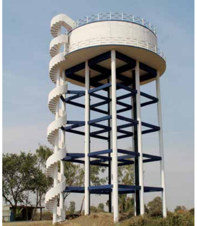
3.6 Lakhs Ltr Capacity Break Pressure Tank (BPT) at Buldhana Water Supply Scheme, in Maharashtra
