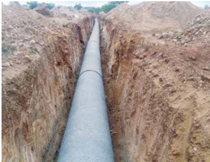
600 mm dia BWSC pipeline laying at Kushtagi MI&GWDD project, in Karnataka.
