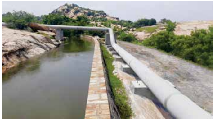
800 mm dia MS Pipeline for canal crossing for Alampalayam project, in Tamilnadu.
