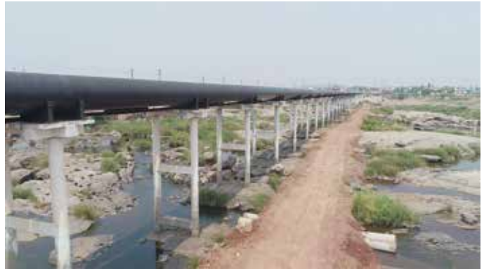
1600 mm dia MS pipeline laying for KPCL Bellary project for a length of 700 mtrs on existing bridge for crossing Tungbhadra River at Hospet, in Karnataka
