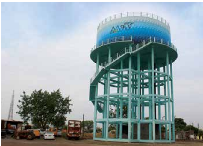
1000 KL Overhead Tank at Jora in Augmentation of Raipur Water Supply Scheme, in Chhattisgarh.
