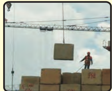
PILE LOAD TESTING
