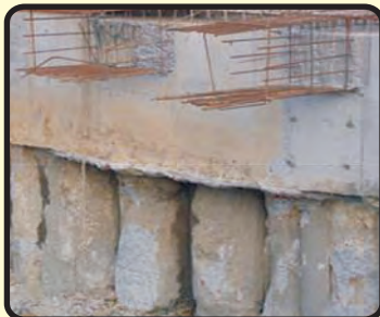
CONTINGUOUS BORED AND SECANT PILE WALLS
