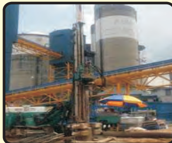
MICRO PILES AND GEOTECHNICAL WORKS
