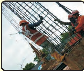
BORED CAST IN PLACE CONCRETE PILES
