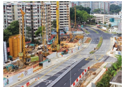
THOMSON LINE - HAVELOCK STATION
