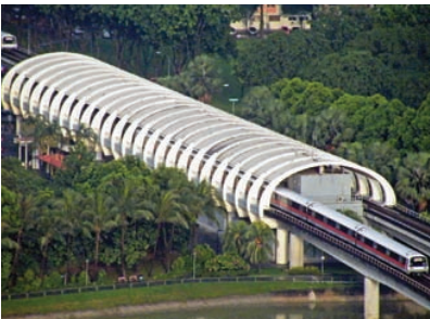
KALLANG MRT STATION
