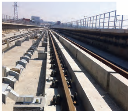
80 km ballastless track Delhi Metro
