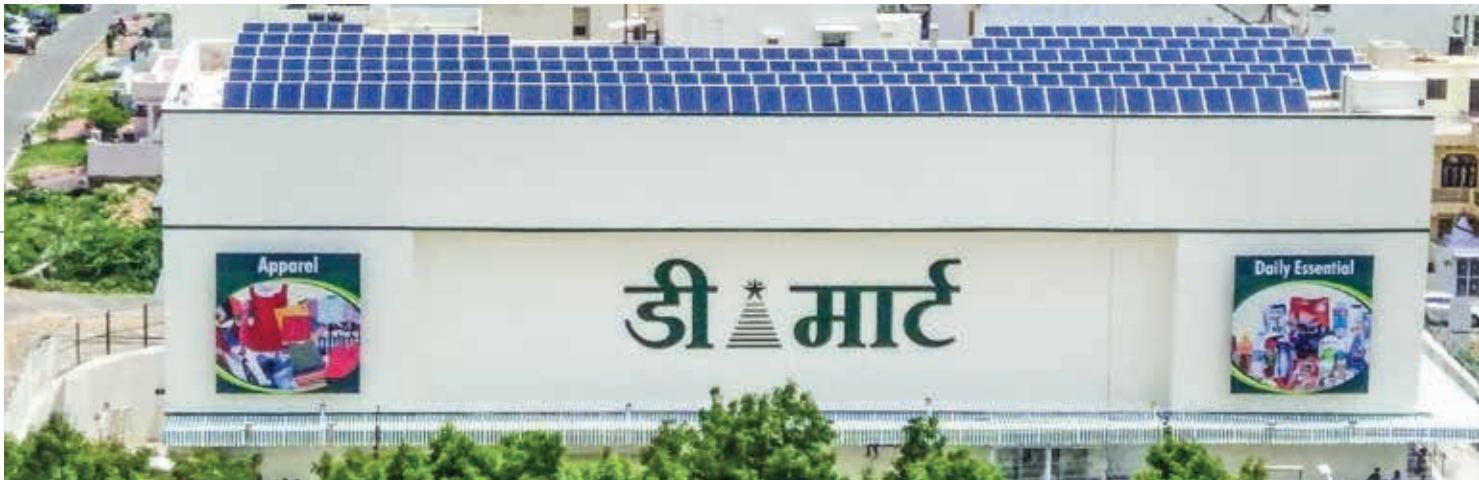
Rooftop Solar Panels
